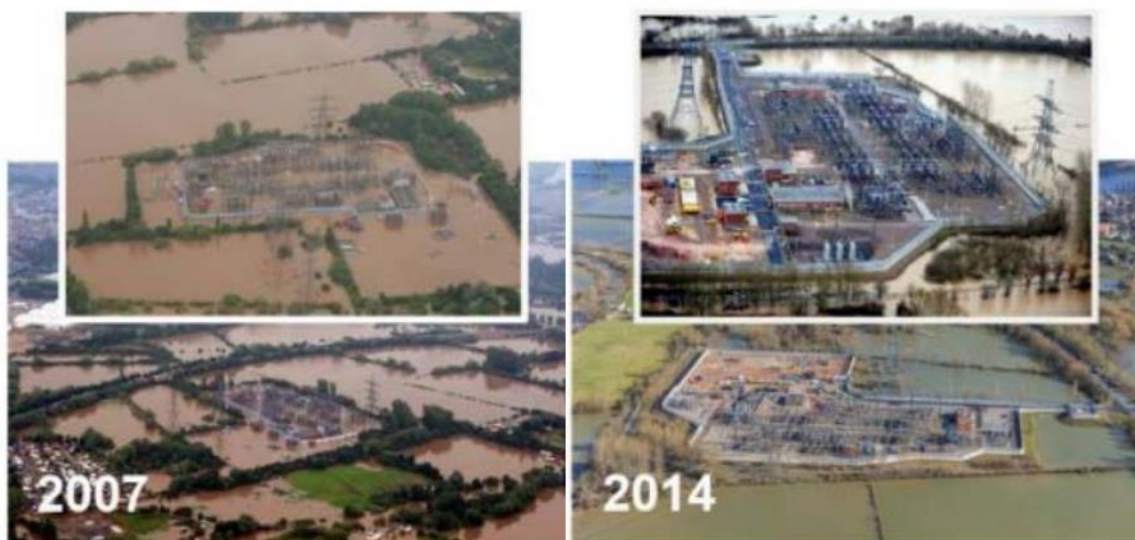
Figure 2: Walham substation flood defences
