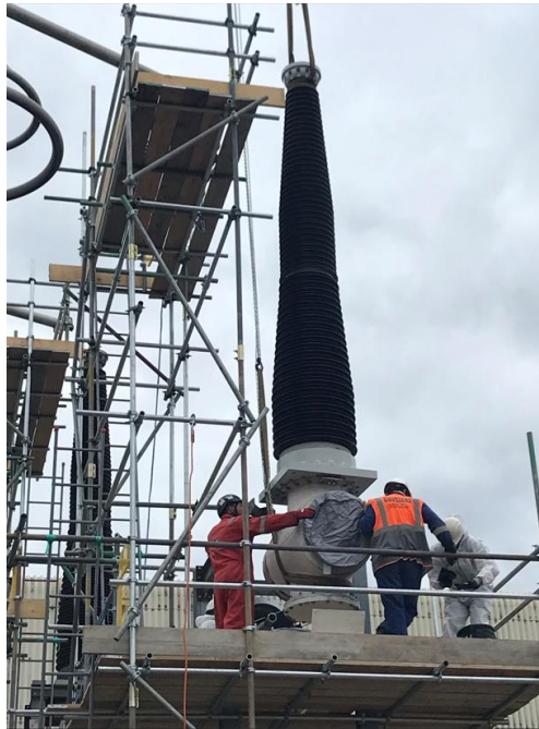
Figure 7.7: Gas to air bushing replacement
