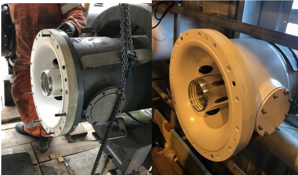
Figure 7.6: 400kV Gas Zone Refurbishment
