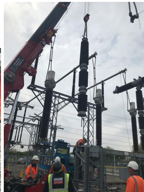
Figure 7.5: Site delivery phase of 400kV Air Insulated Substation Gas Circuit Breaker Repair
