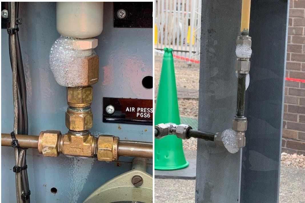
Figure 6.10: Use of leak detection spray
