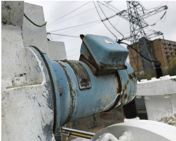
Figure 6.7 (Left): [REDACTED] GIS at [REDACTED] showing evidence of corrosion
