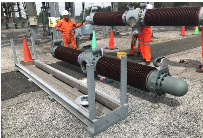
Figure 7.5: Site delivery phase of 400kV Air Insulated Substation Gas Circuit Breaker Repair
