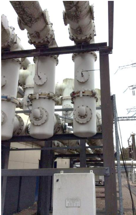
Figure 6.7 (Left): [REDACTED] GIS at [REDACTED] showing evidence of corrosion
