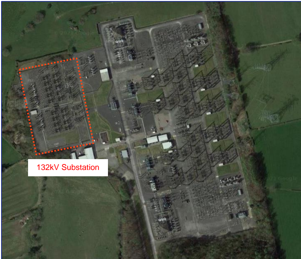
Figure 2 – Aerial view of Cellarhead substation
