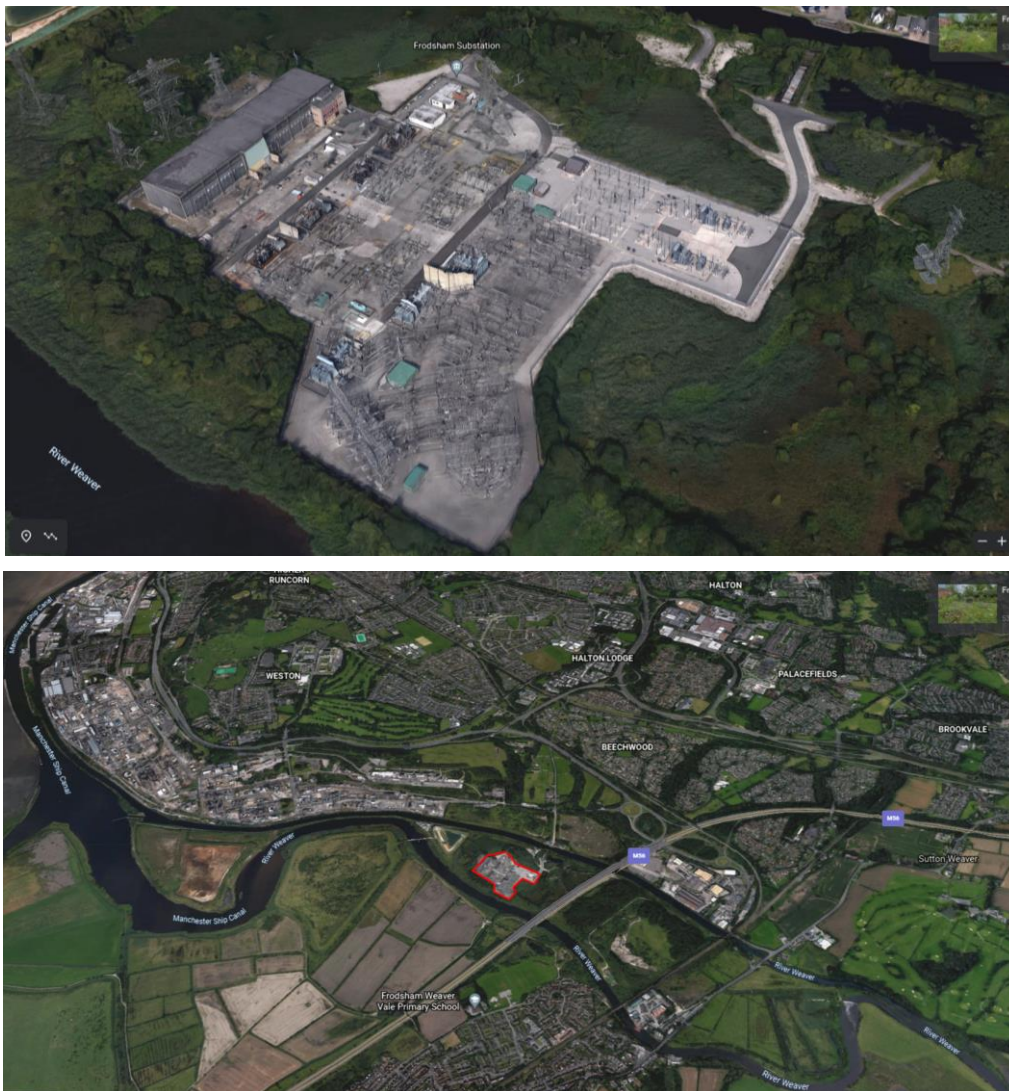
Figure 2 – General view of Frodsham 400kV Substation
