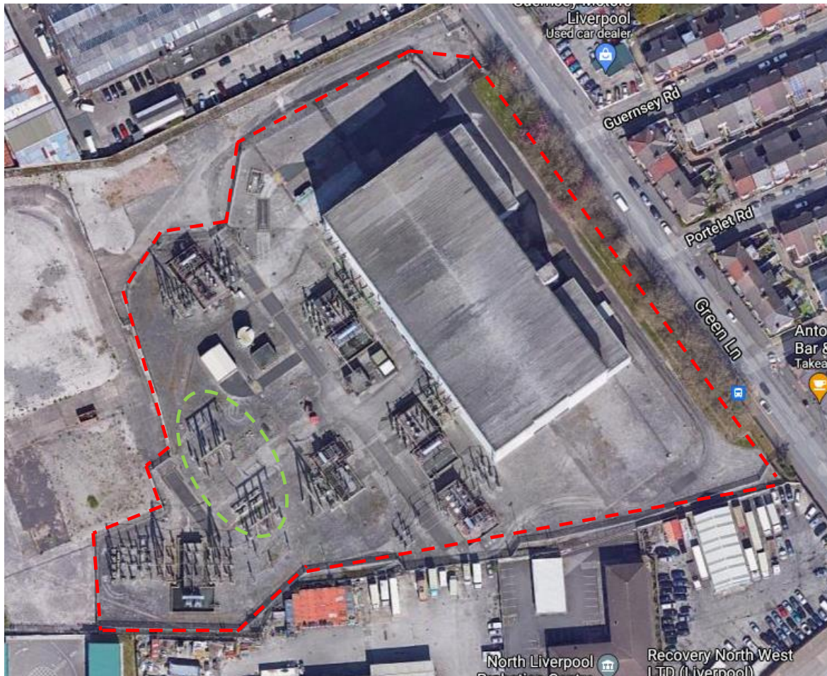
Figure 5 – Location of Lister Drive – Birkenhead circuit overhead busbar section
