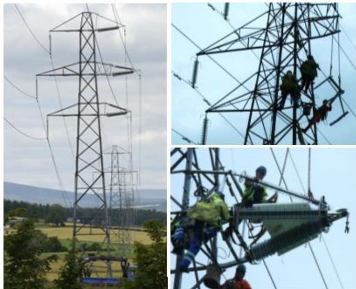
Figure 33 – Installation of RICAs on SHETL network
