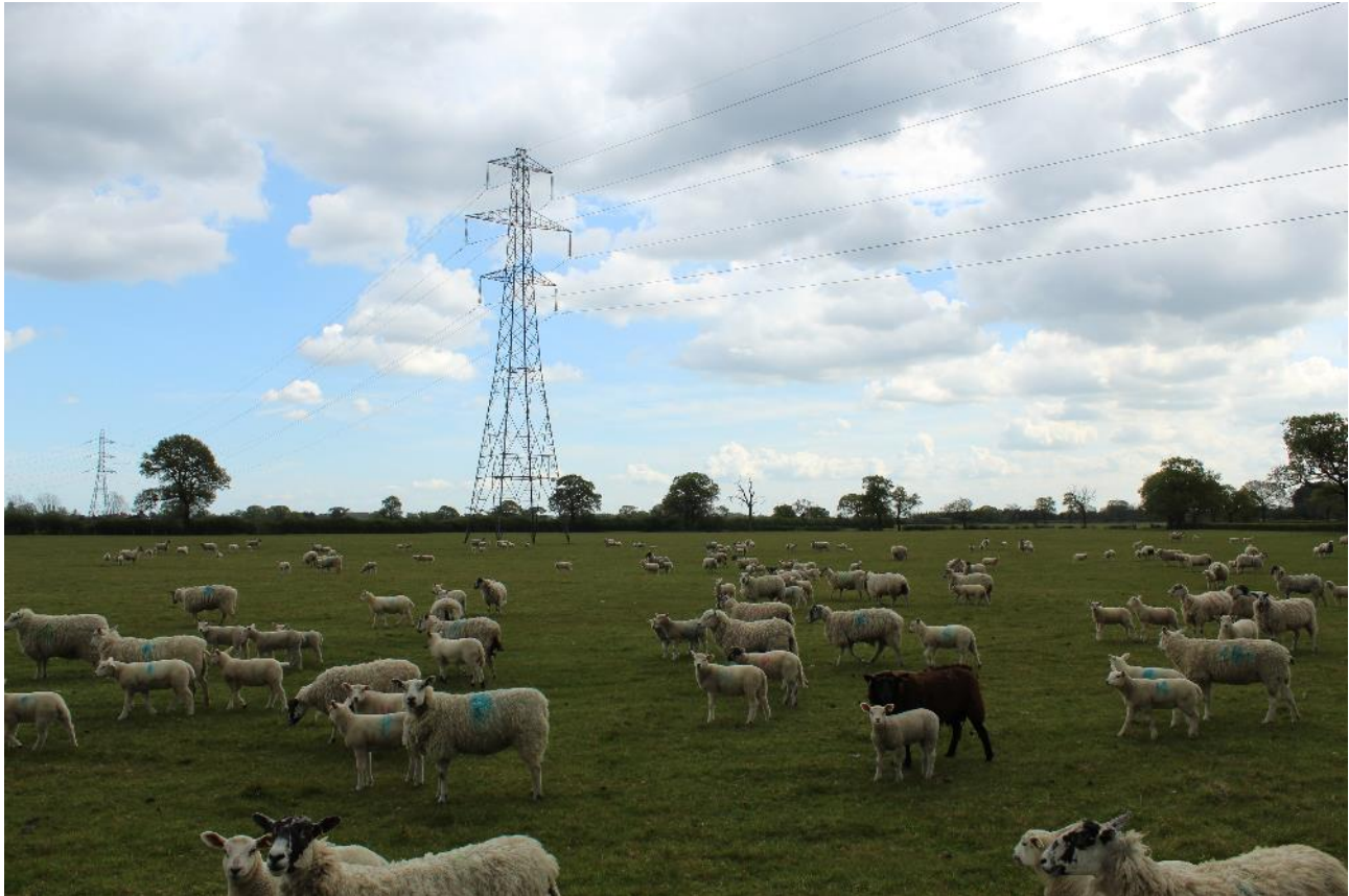
Image 2 - Site of cropmark around pylon XCP 008
