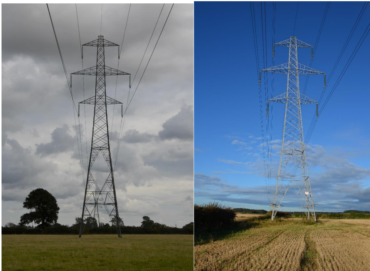
Figure 3.1b – Example of single conductors (left image) and twin conductors (right image)
