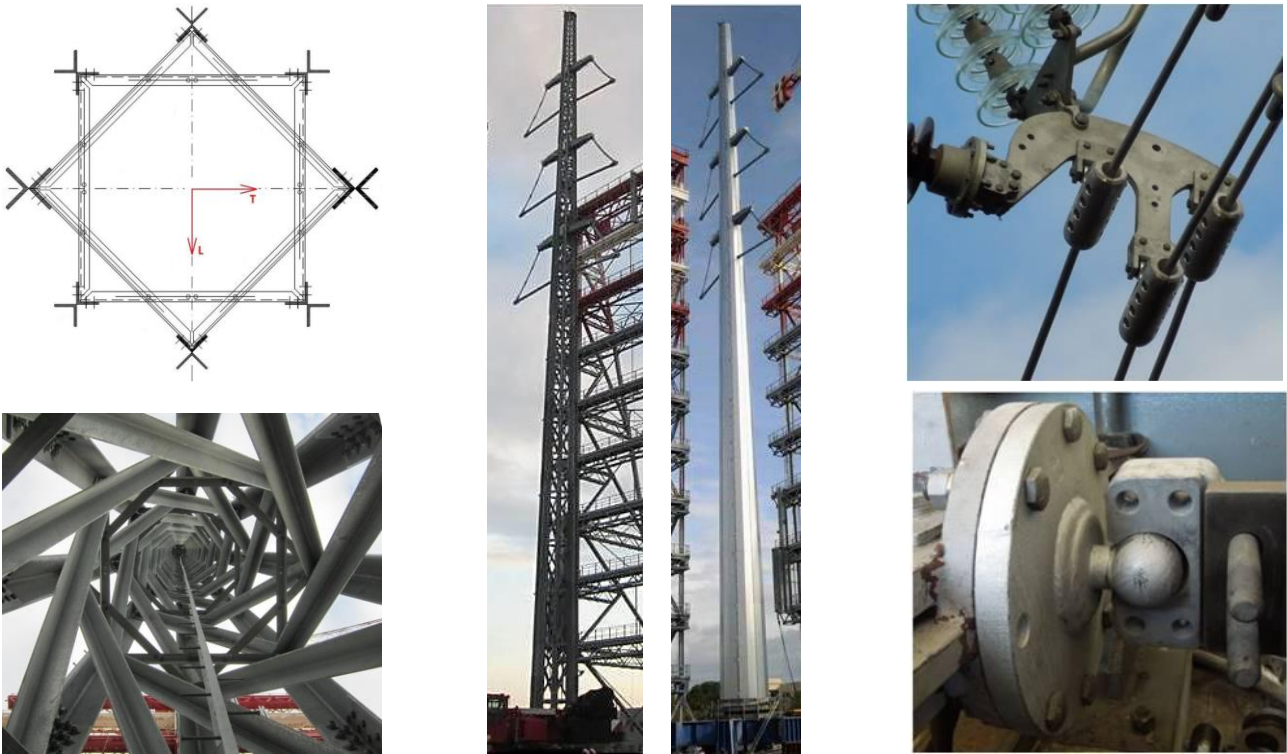
Figure 2.14 - Vitruvio tower main members connections and internal view (left), assembled tower with and without external cover (middle), suspension clamp and ball joint (right). [15]
