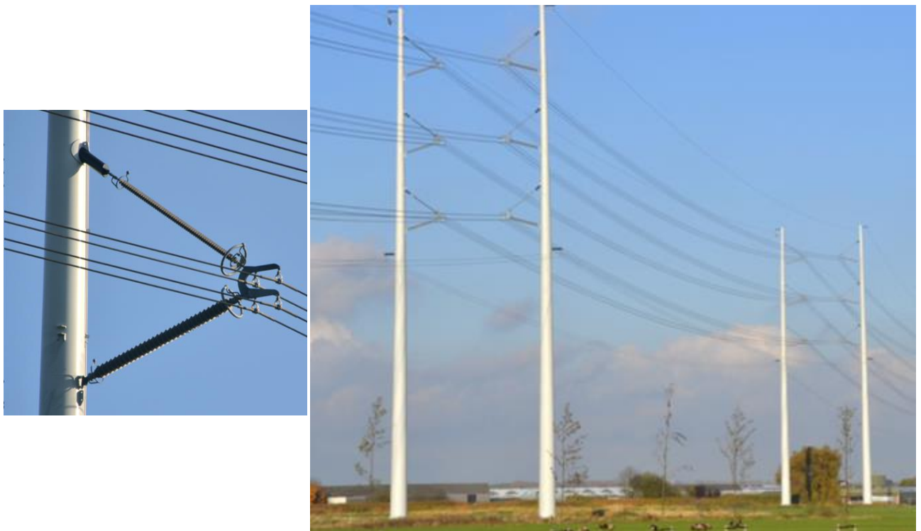
Figure 2.15 - Wintrak ICA (left) and Wintrak towers (right) [16]
