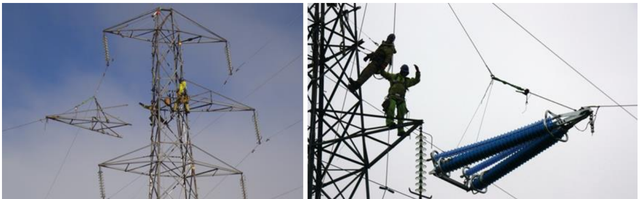
Figure 6.3 - Removing the steel cross-arm (left) and raising the insulating cross-arm (right) [4]
