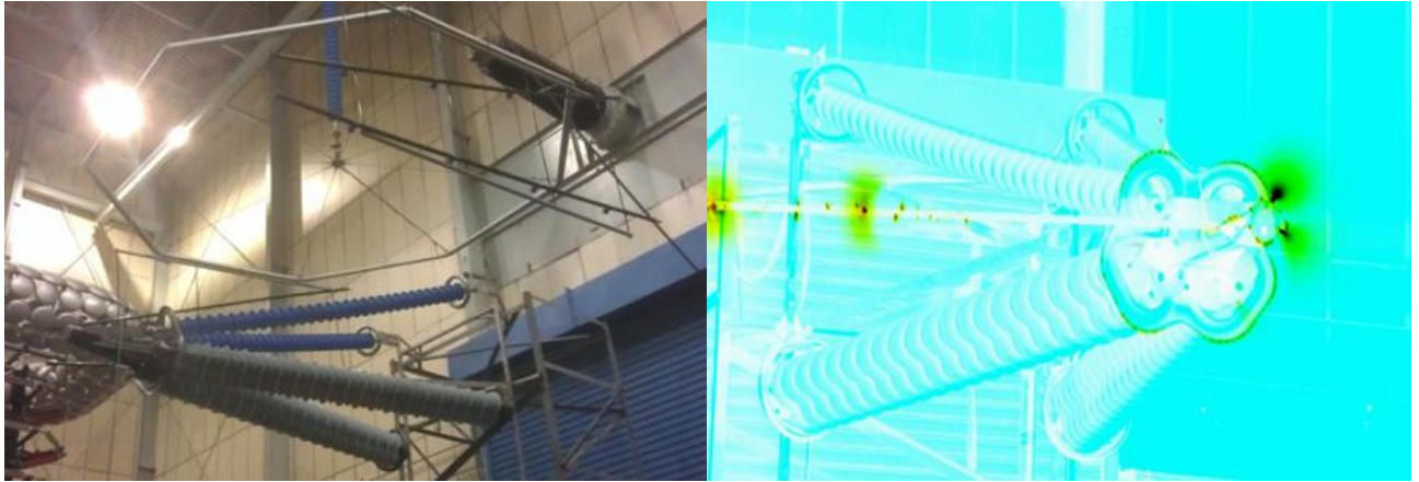
Figure 6.2 - Wet switching impulse withstand voltage test using bespoke spray system (left) and Corona Extinction test (right)
