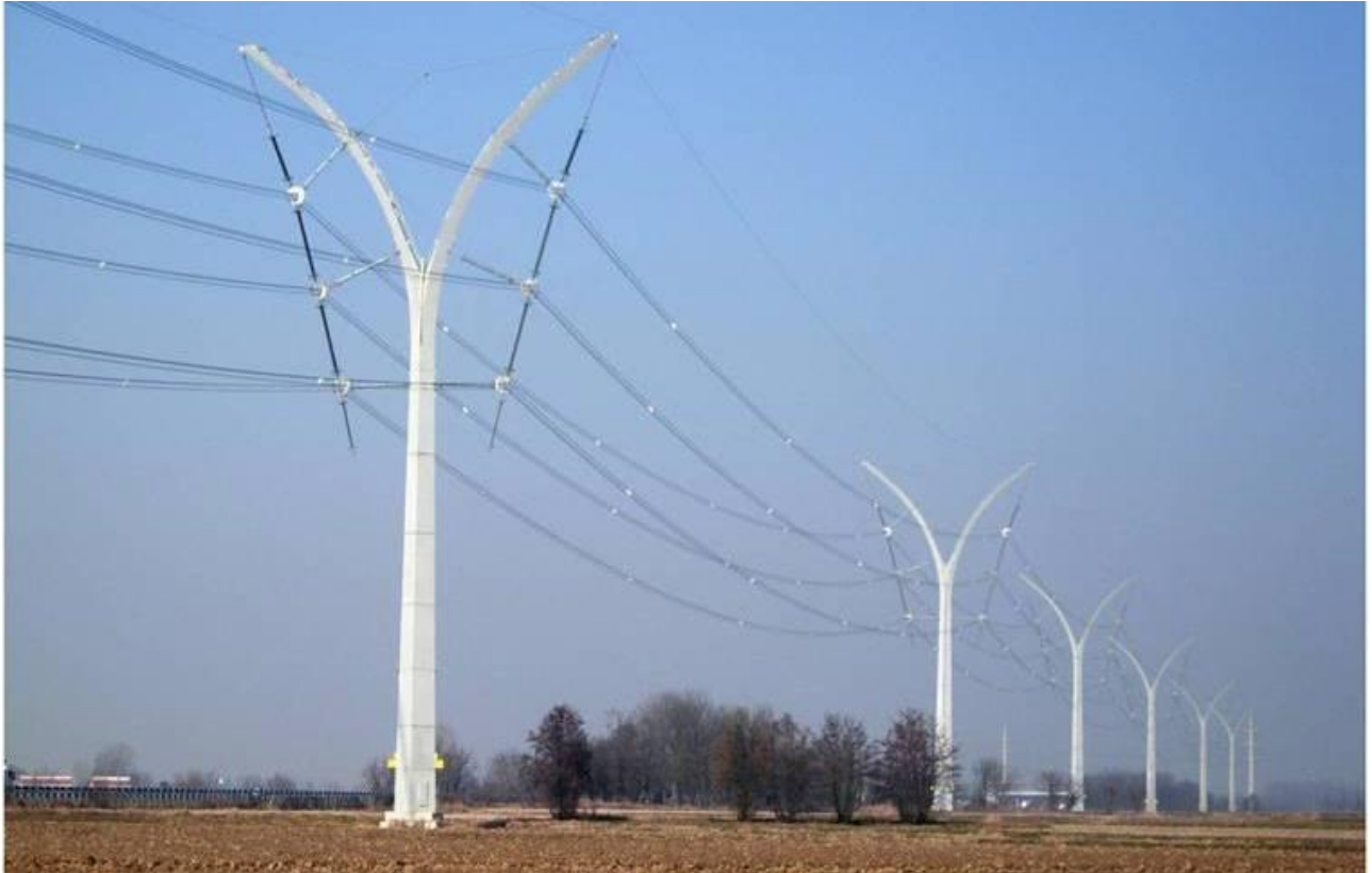
Figure 2.19 - Trino – Lacchiarella “Germoglio” towers in operation [20]
