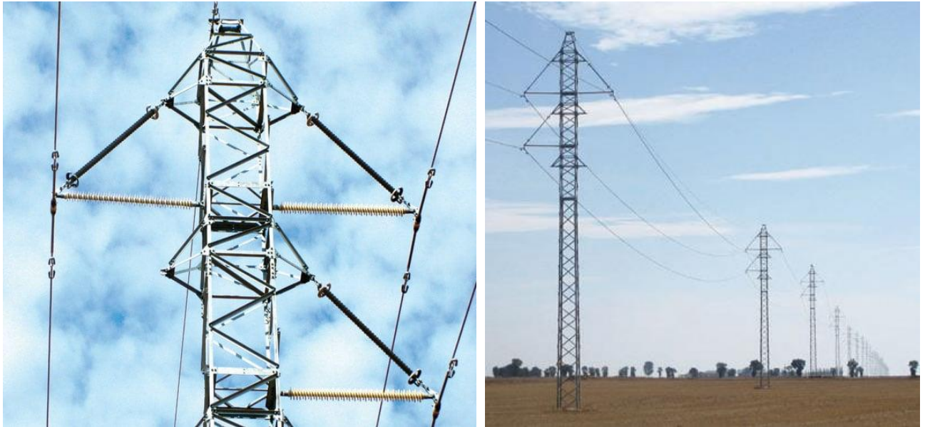
Figure 2.12 - Horizontal Vee ICAs (left) and compact line running through agricultural land (right) [14]
