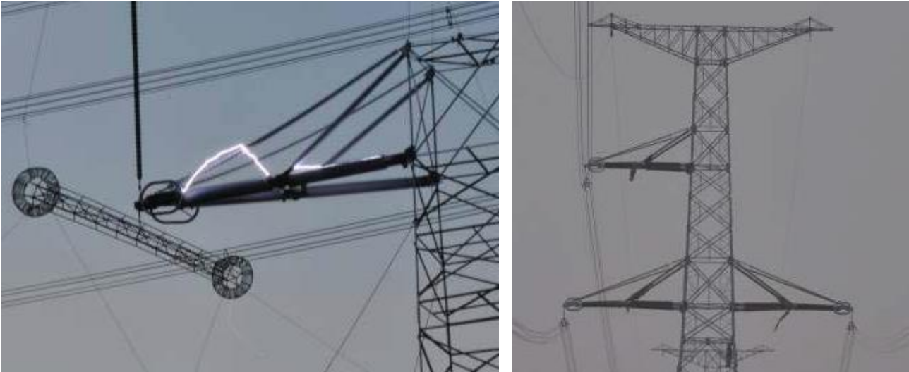
Figure 6.7 - Switching impulse test (left) and ICAs installed on a live line (right)
