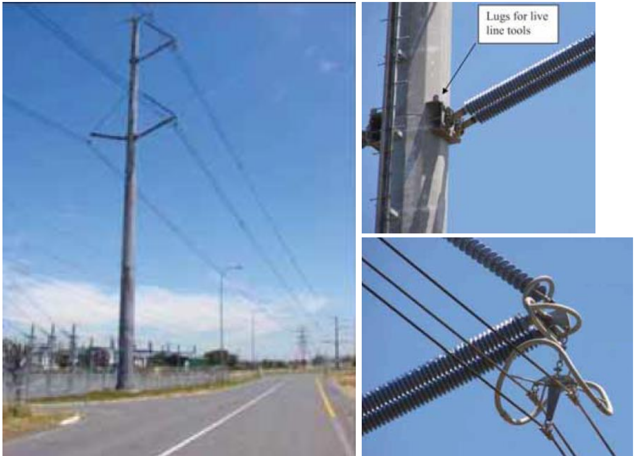
Figure 2.20 - 531A single pole suspension steel mast and double braced post insulator [21]
