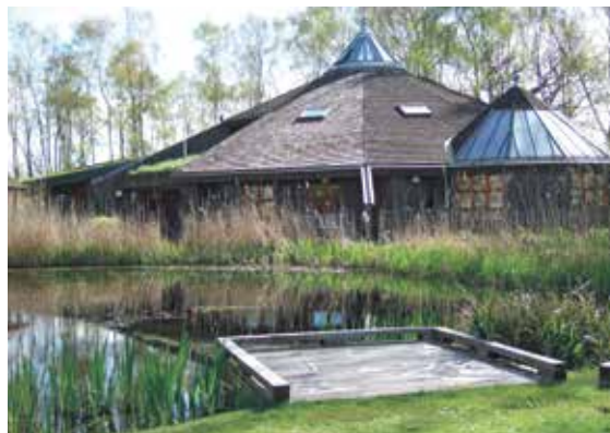
Above: Young and old will find out more about the countryside when they visit Bishops Wood Below: The new eco centre built with sustainably sourced wood has a turf roof and reed bed sewage treatment system
