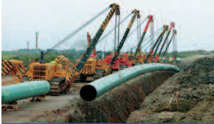
Pipes are lowered into the trench
