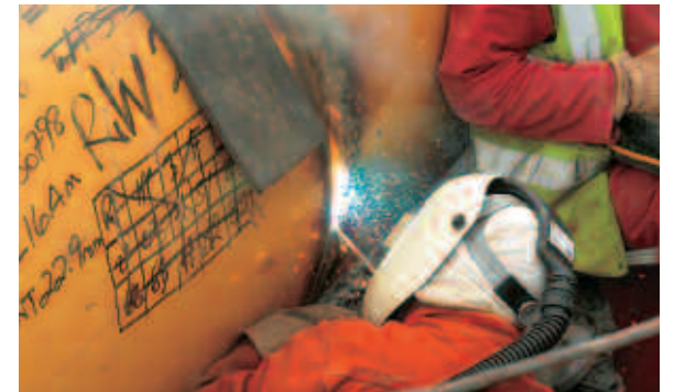
Welders join sections of the pipes
