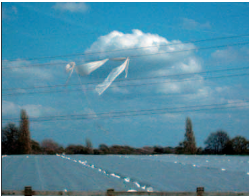
The sheeting caught up in the overhead line on the Daines-Deeside circuit which, fortunately, was out of service
