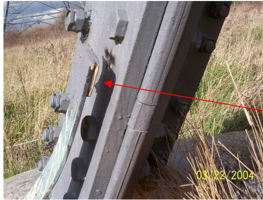
Figure 8.4 - Example Defective Earth Tape Connection
