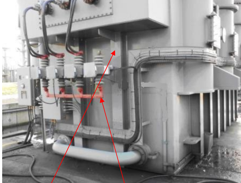
Figure 7.2b - Defective or missing neutral earth connections between the Equipment star point and the Main Earth System
