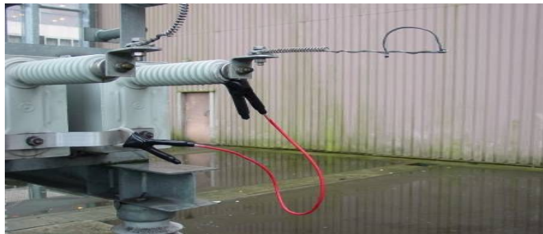
Figure 8.3A – Applying the Clip-on Short-Circuiting Lead
