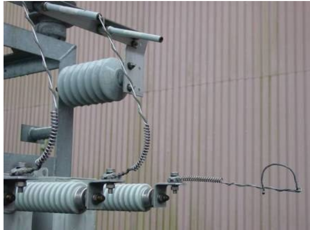
Figure 5.2B - Identifying an Externally Fused Capacitor with a Fuse Operated
