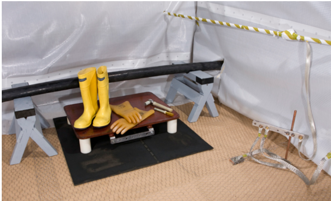
A photograph of a bay set up for Insulated Working .
