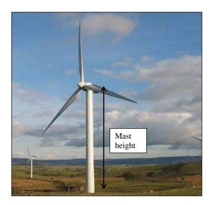
Based on the study, the appropriate exclusion zone (distance from base of the wind turbine mast to the edge of the pipeline) has been identified as 1.5 times the turbine mast height.
