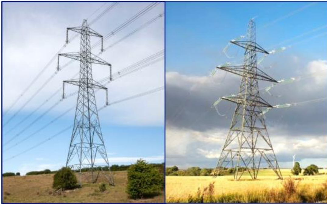
Figure 2-2: Suspension Pylon (Left) and Angle Pylon (Right)
