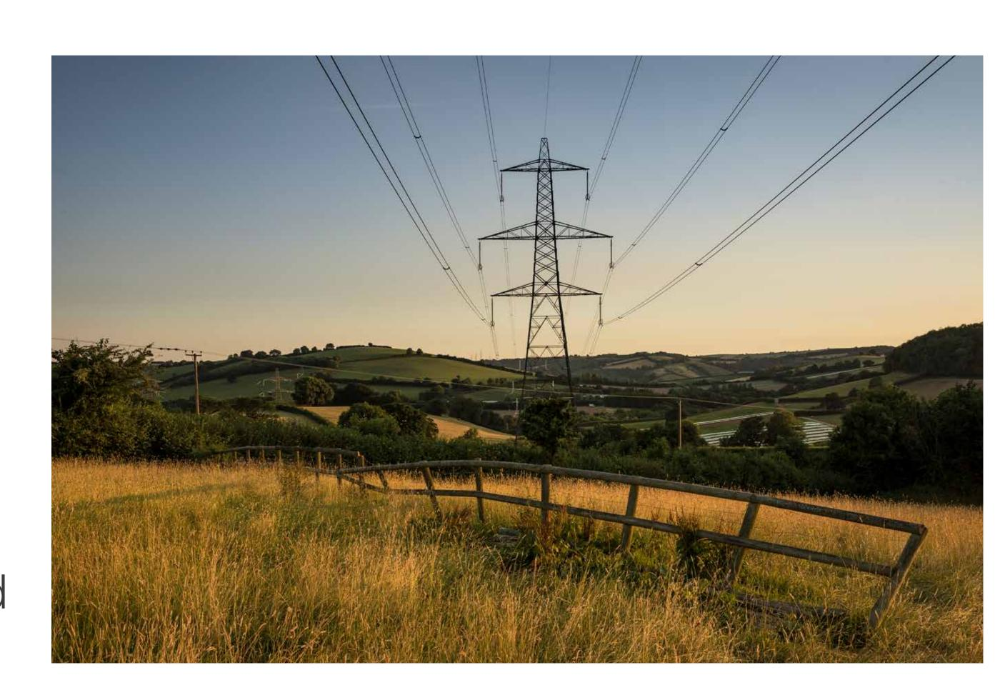
Like most overhead lines owned and maintained by NGET, the project will carry a voltage of 400 kV. These are typically around 50 metres in height, with approximately three pylons per kilometre on a straight section of corridor, potentially slightly more in places. In some locations, specific constraints such as navigable river crossings, can require considerably taller pylons to ensure safe electrical clearance from the overhead lines to the activities below them.
