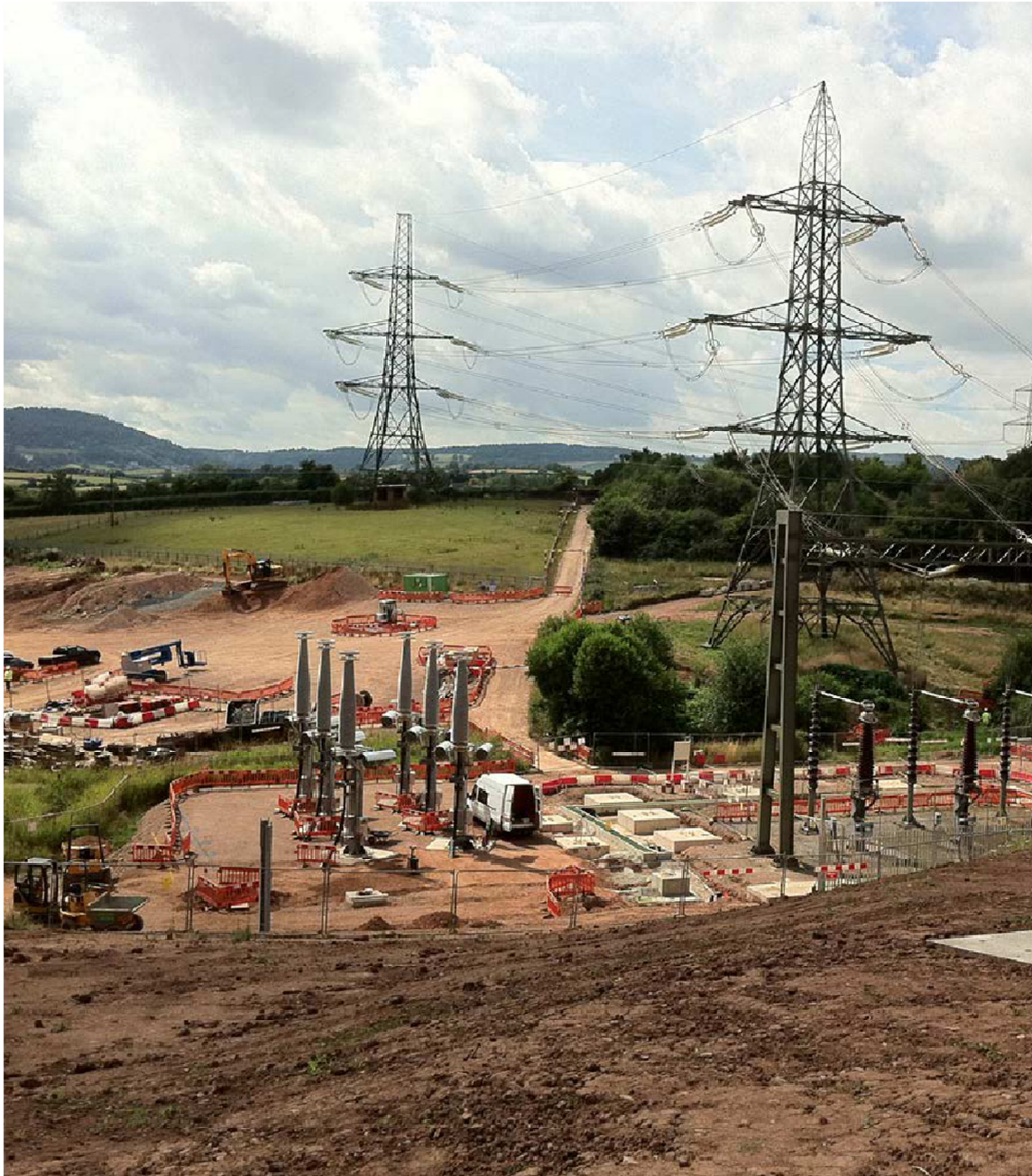
The undergrounding of electricity cables at Ross-on-Wye
