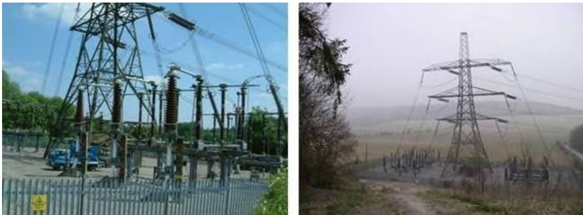
Figure C.5 – Cable Sealing End Compounds
