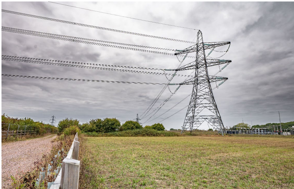
Image 2.1 Typical suspension steel lattice pylon
