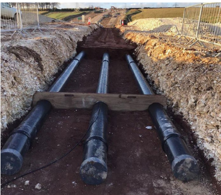
Constructing underground cable
