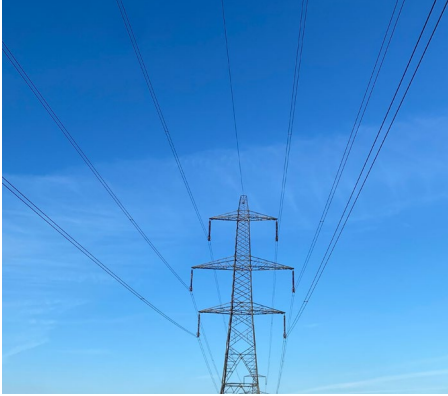
Example of a 400 kV steel lattice pylon
