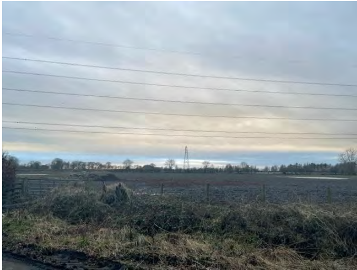
Distant view of tower on T route
