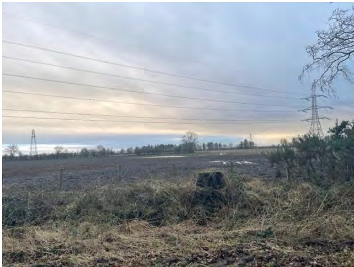
View of tower on T Line (Order Line) in the context of Tower on AL line (existing deed Line)
