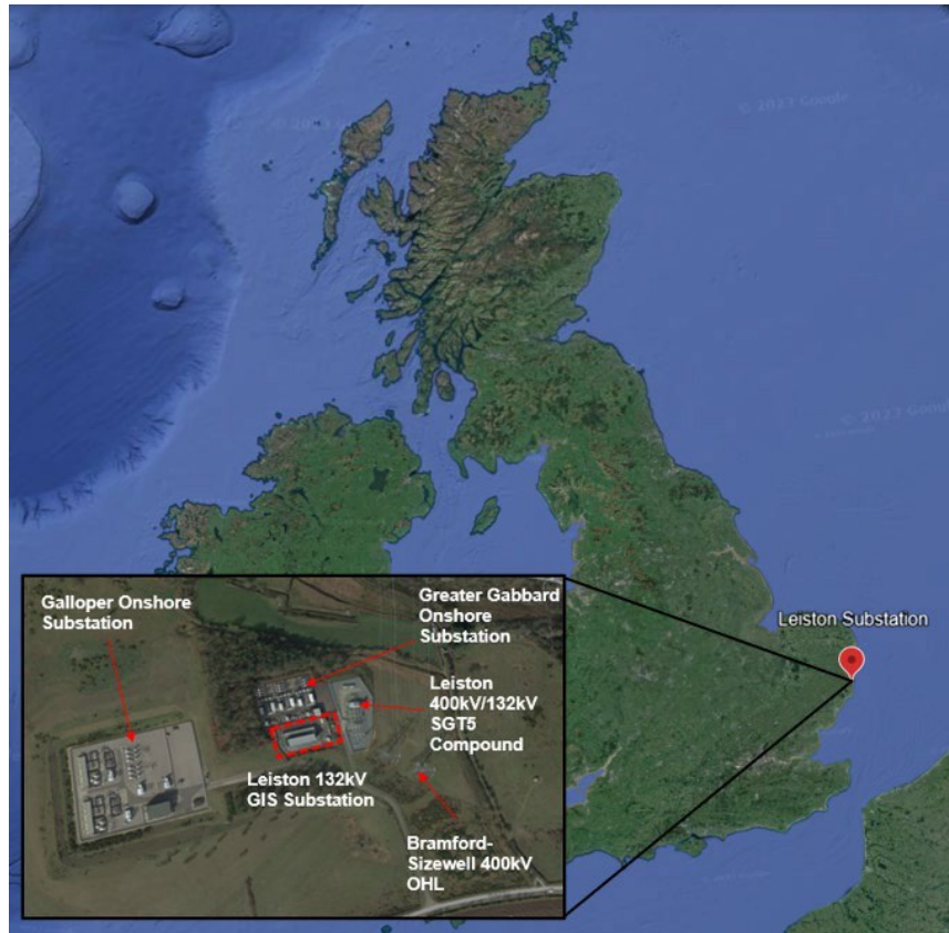
Figure 2 – Aerial view of Leiston substation
