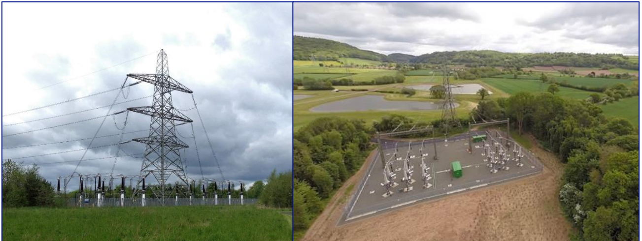
Figure 2-6 – Example 400 kV Sealing End Compounds
