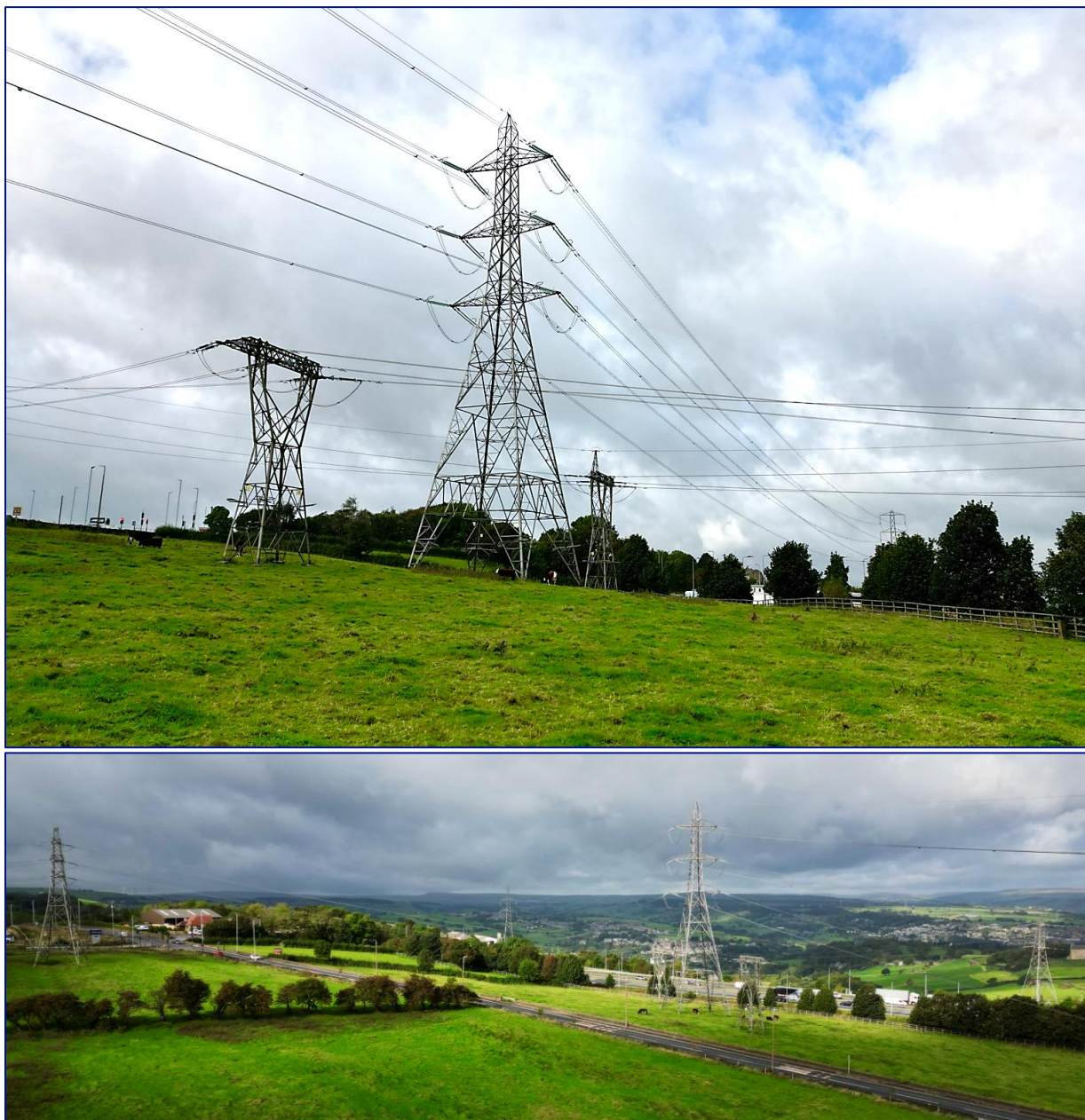
Figure 5-17 – Examples of an Overhead Line Duck Under
