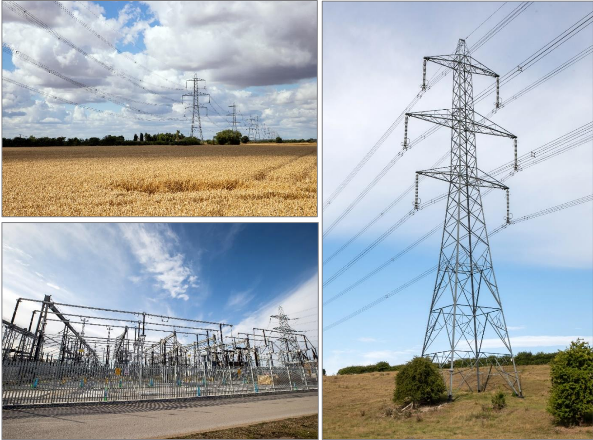
Figure 1-1 – Example Images of NGET’s Transmission System
