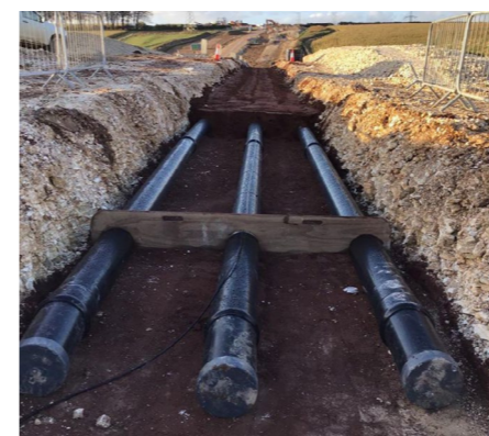
Constructing underground cable
