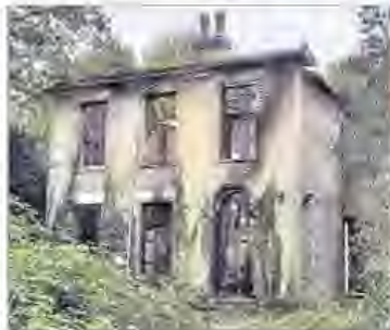
Rose Hill in Ash, after the fire
