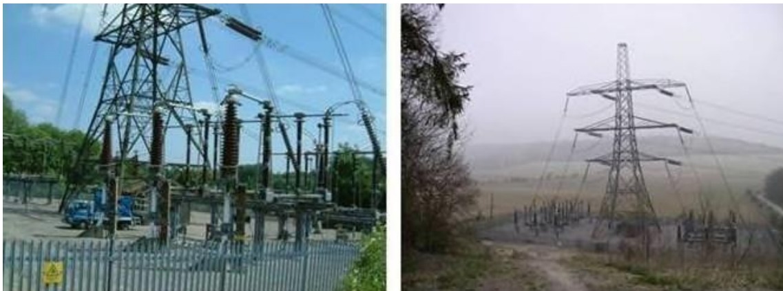
Figure C.5: Cable Sealing End Compounds
