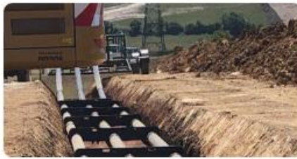
VIP project under construction
