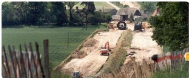
Newbury Nunthorpe VIP undergrounding
