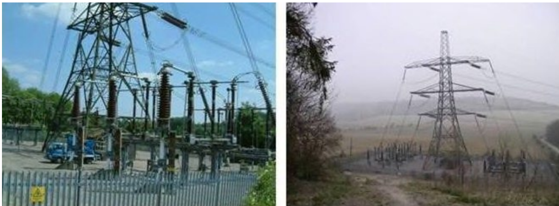
Figure C.5: Cable Sealing End Compounds
