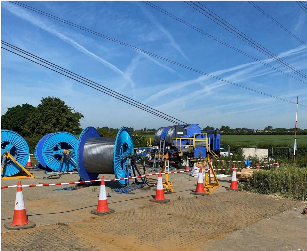
Layout of an Equipotential Zone (Ensure Positioned to Maximise Clearance to Adjacent Live Circuit)
