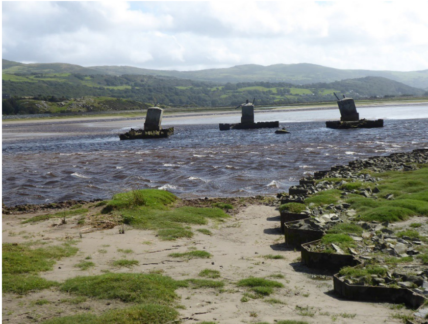
Plate 15.8: Site 4ZC030 remaining pylon foundations located within the estuary channel
