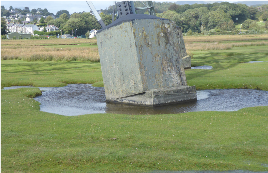
Plate 2.9: Pylon 4ZC031 Chimney and Muff
