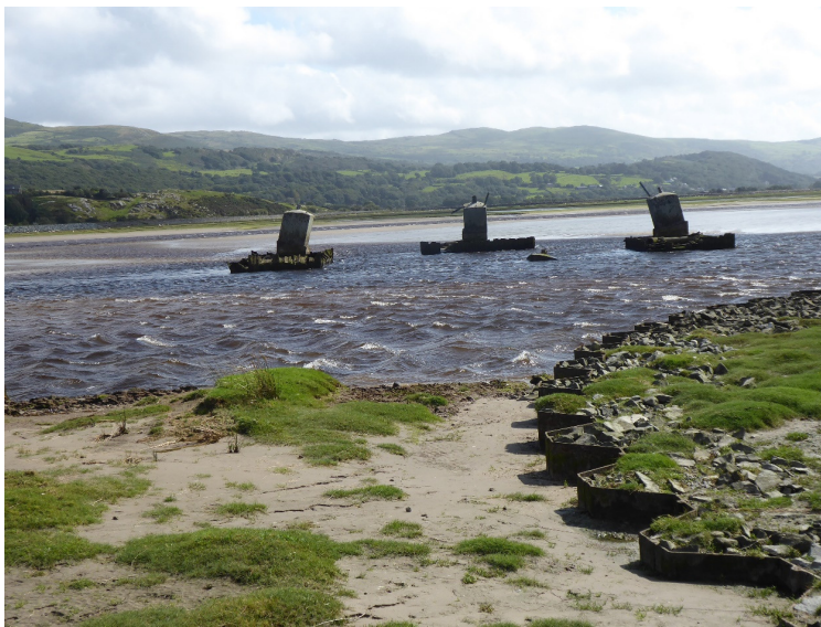
Plate 2.3: 4ZC030 foundations in the estuary (2019)
