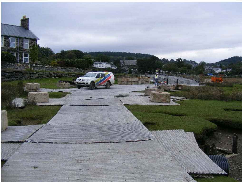
Plate 2.12: Photograph of trackway for previous works on Pylon 4ZC030R
