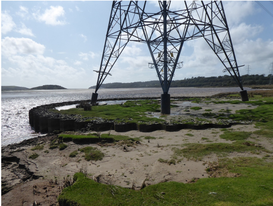
Plate 2.6: 4ZC030R Foundations and cofferdam at the edge of the estuary channel (2019)
