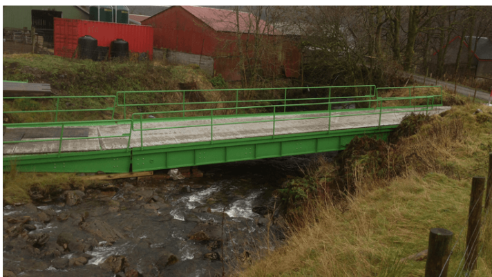
Figure 3-14 An example of a vehicular bridge
