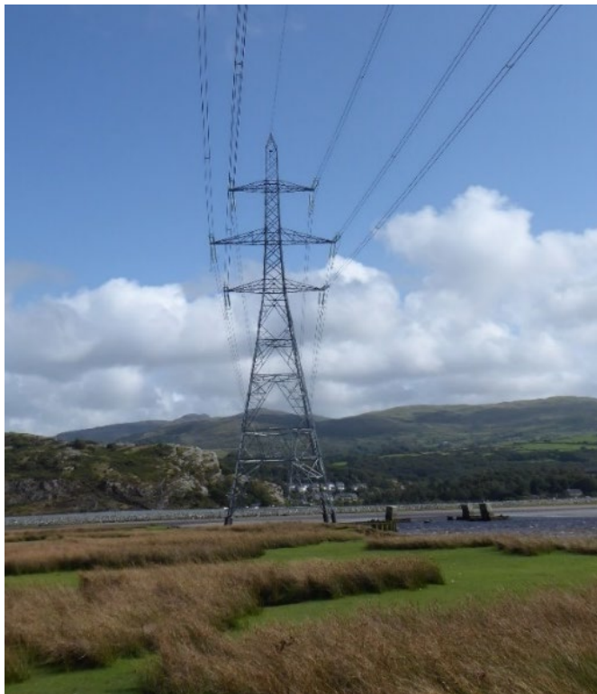
Figure 3-2 4ZC030R Replacement pylon on the edge of the saltmarsh (2019)
