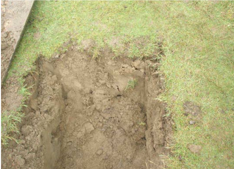
Figure 4-8 Trial pit at edge of saltmarsh, TP04 (Norwest Holst, 2009)
