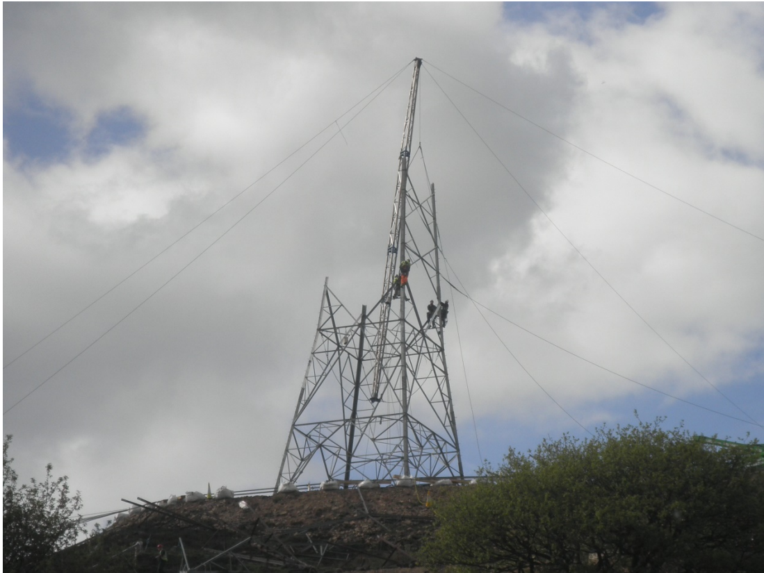
Figure 3-9 Example of a derrick being used to dismantle a pylon
