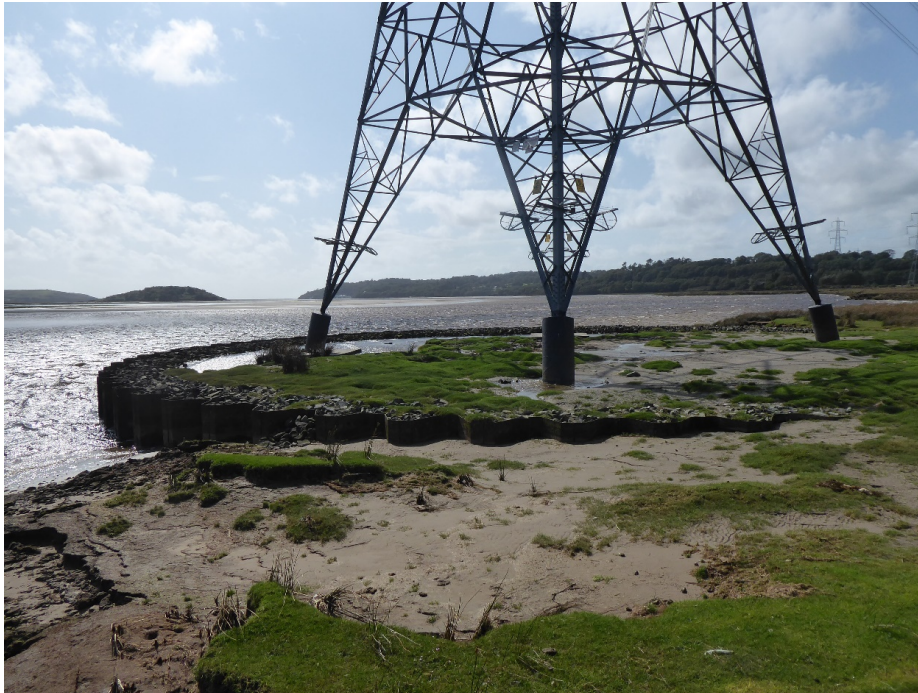
Figure 3-5 4ZC030R Foundations and cofferdam at the edge of the estuary channel (2019)
