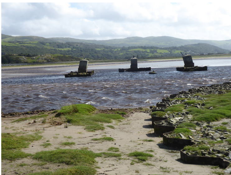
Figure 3-1 4ZC030 foundations in the estuary (2019)
