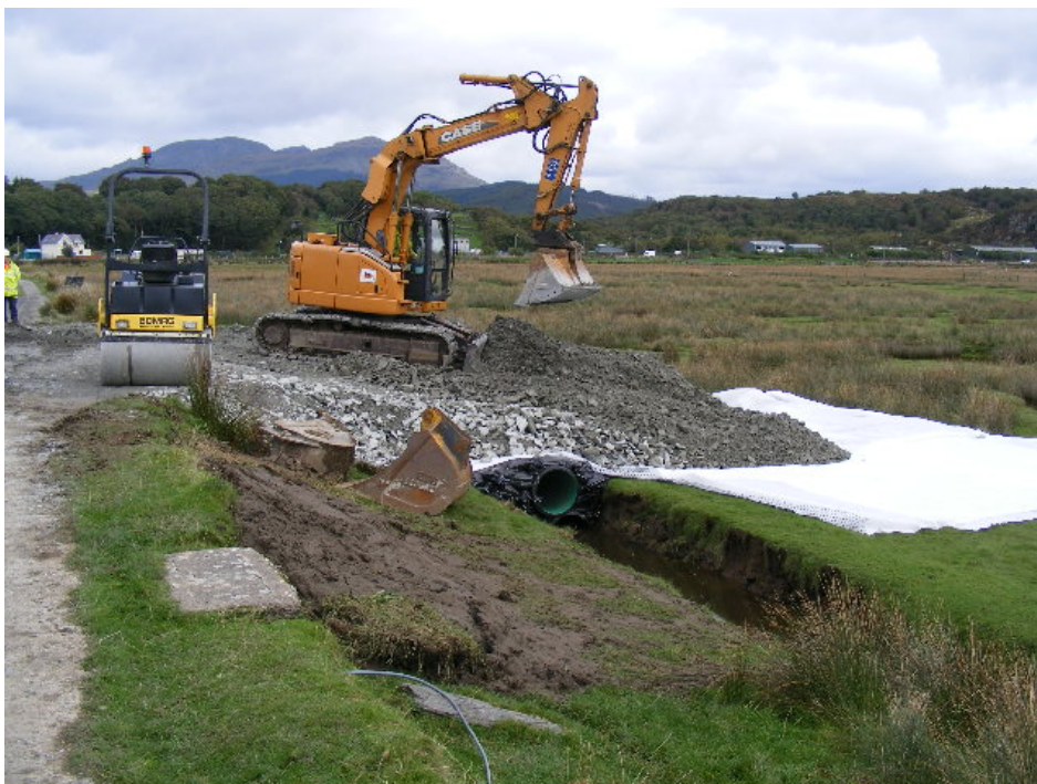
Figure 3-12 Construction of a similar culverted ramp along the existing track in 2013
