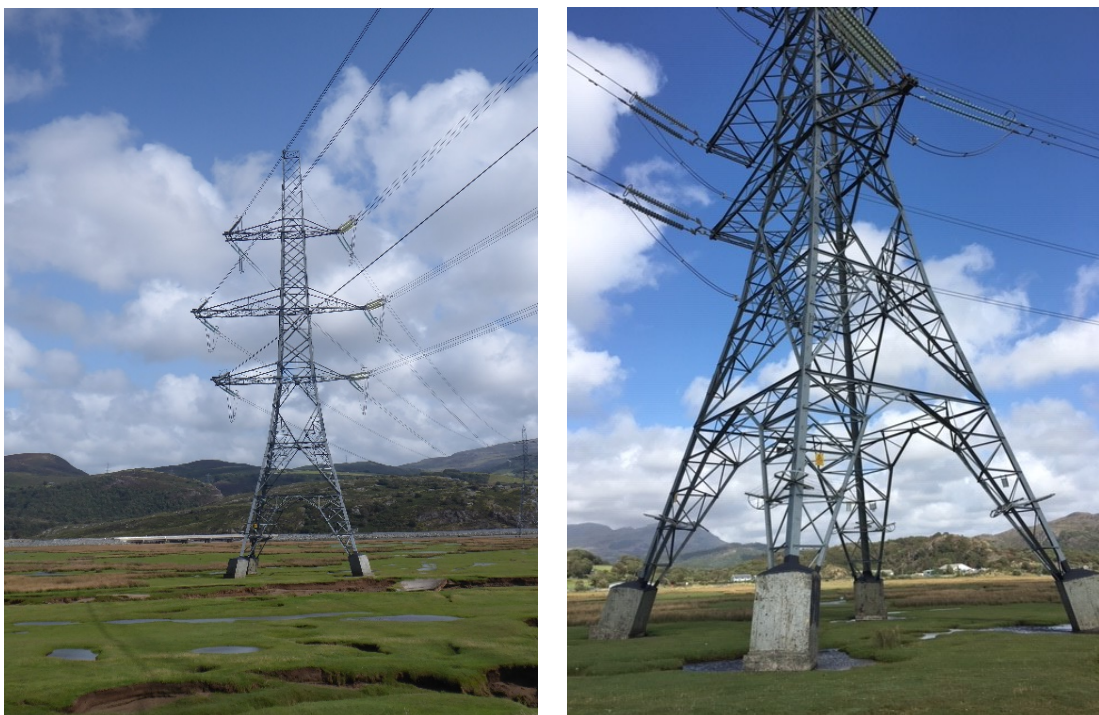
Figure 3-6 4ZC031 Pylon on saltmarsh (2019)
