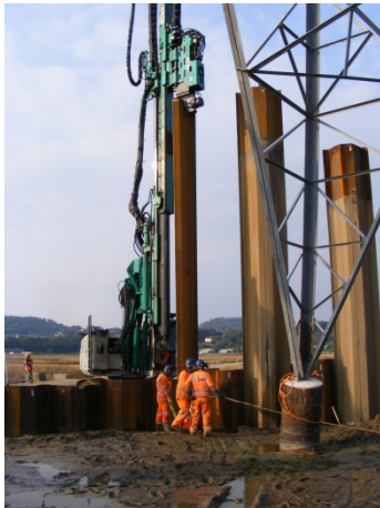
Figure 3-11 Removal of cofferdam sheet piles using leader pile rig
