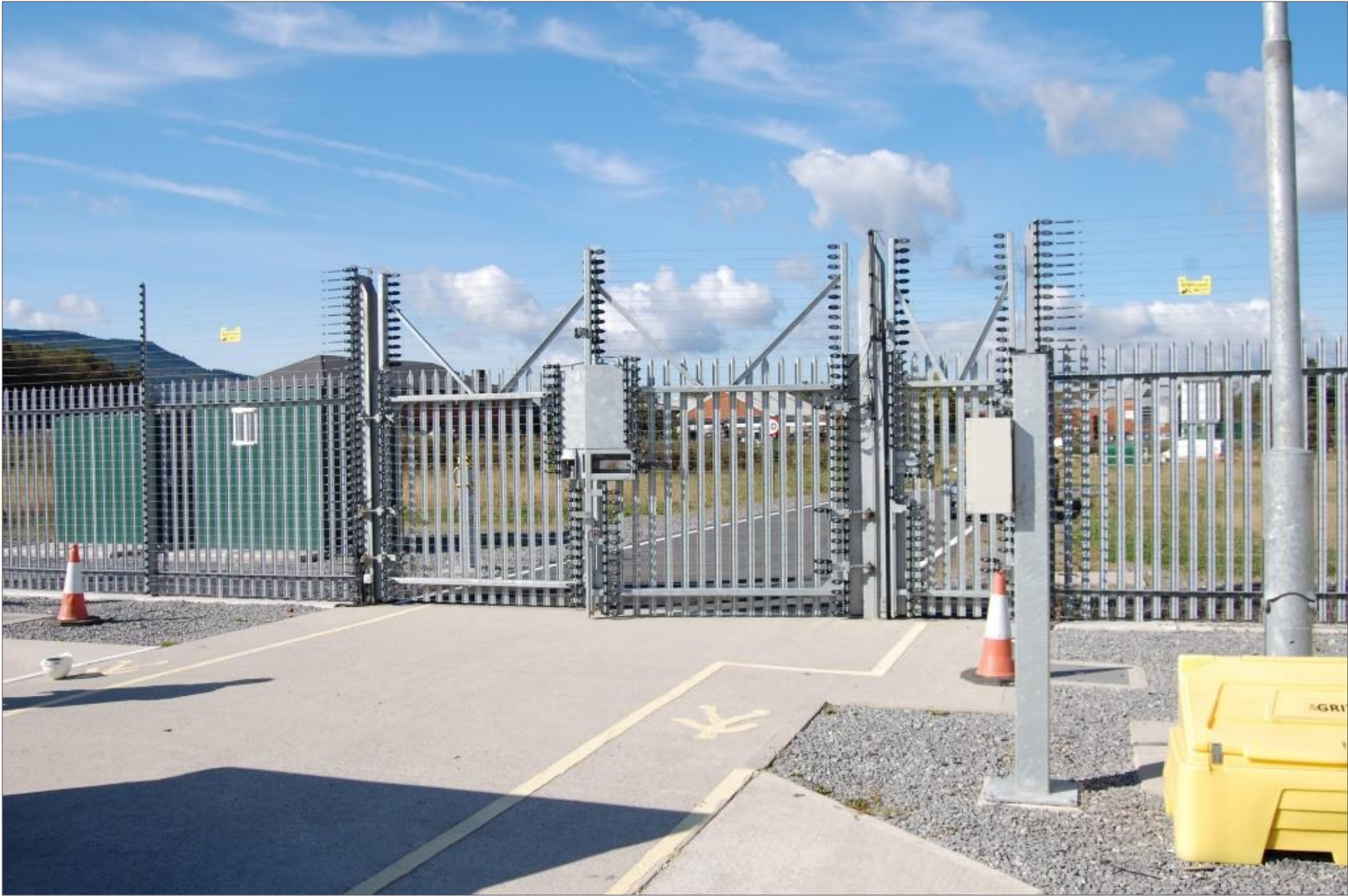
Figure 5.4: Example of palisade security/safety fence and gate
