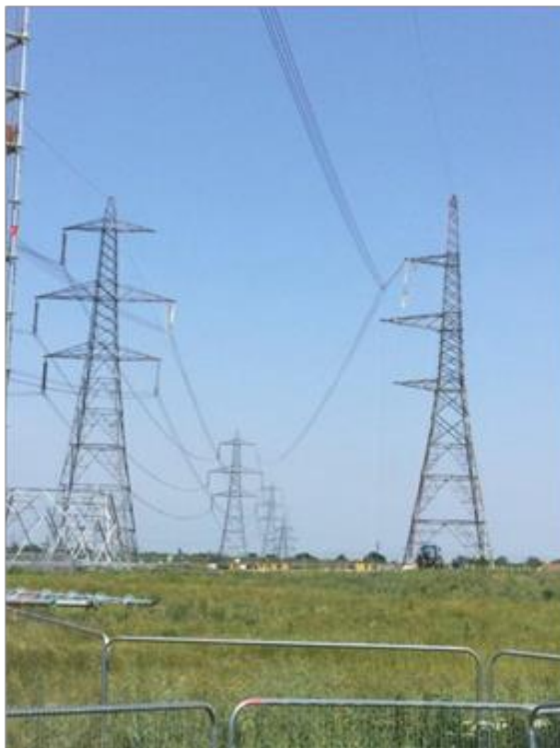
Image 1: Example of a temporary single-circuit overhead line diversion
