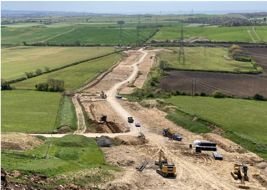
Figure 3.3 – 400kV underground cable swathes
