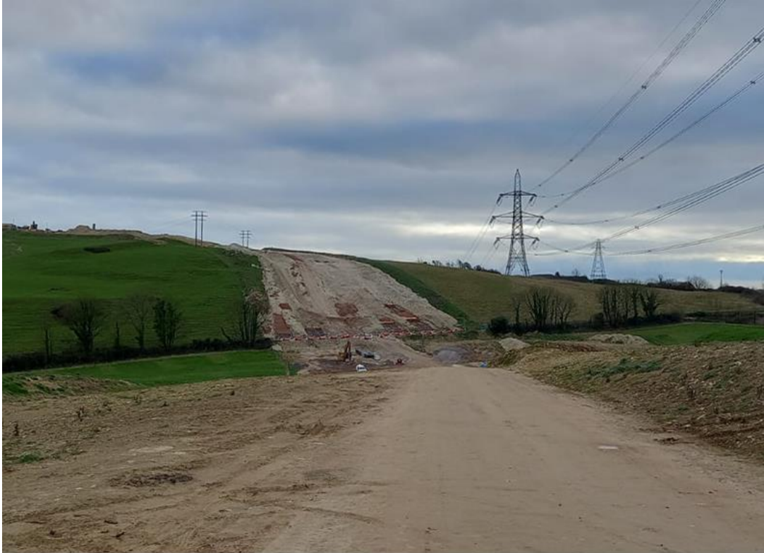
Figure 3.4 – 400kV underground cable swathes
