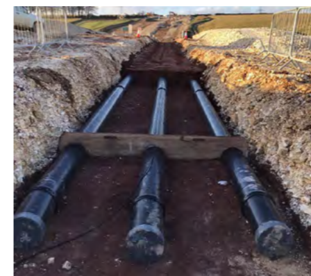
Constructing underground cable
