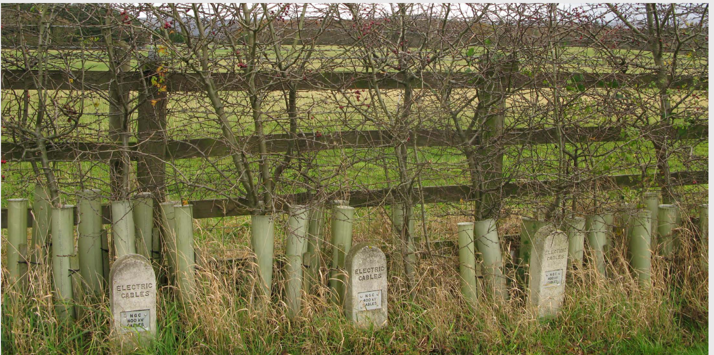
Example of reinstated hedge above underground cables
