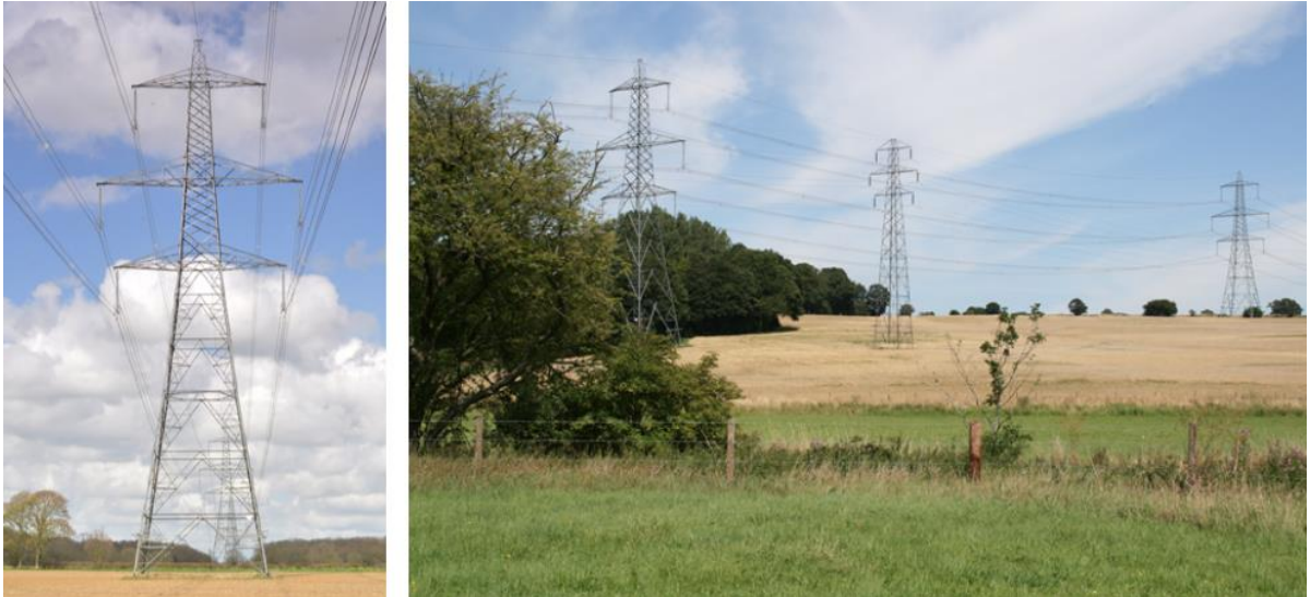
Figure 2.2: Existing 400kV line passing through Hintlesham Woods (left) and both the existing 400kV and 132kV lines near the River Box (right)
