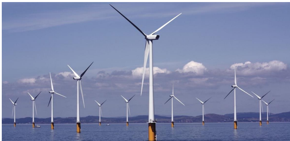
1 One of the increasing numbers of offshore wind farms being built as we move to a renewable based power system.
