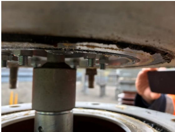
Figure 8 – Photos of leaking LTB145 circuit-breaker
