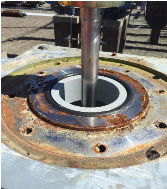
Figure 9 – Photos of leaking FE circuit-breaker
