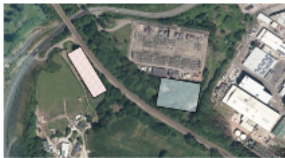
Aerial view: Looking at connection options and potential challenges
