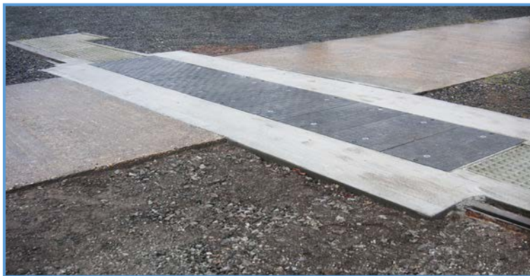
Figure A1: Vehicle trench crossing
