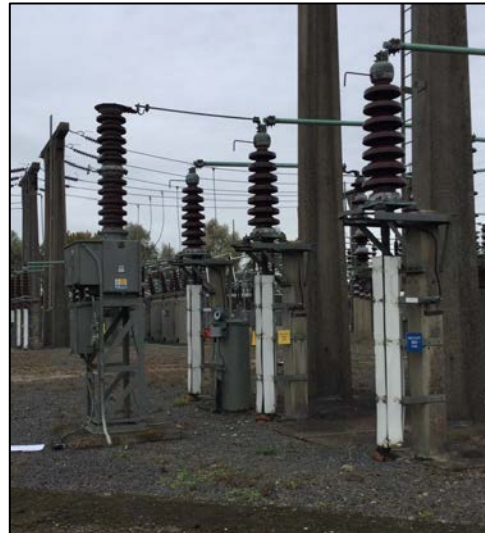
Figure 2 – Single Phase 132kV Capacitor VT at Grendon 132kV Substation
