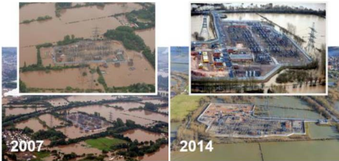
Figure 2: Walham substation flood defences
