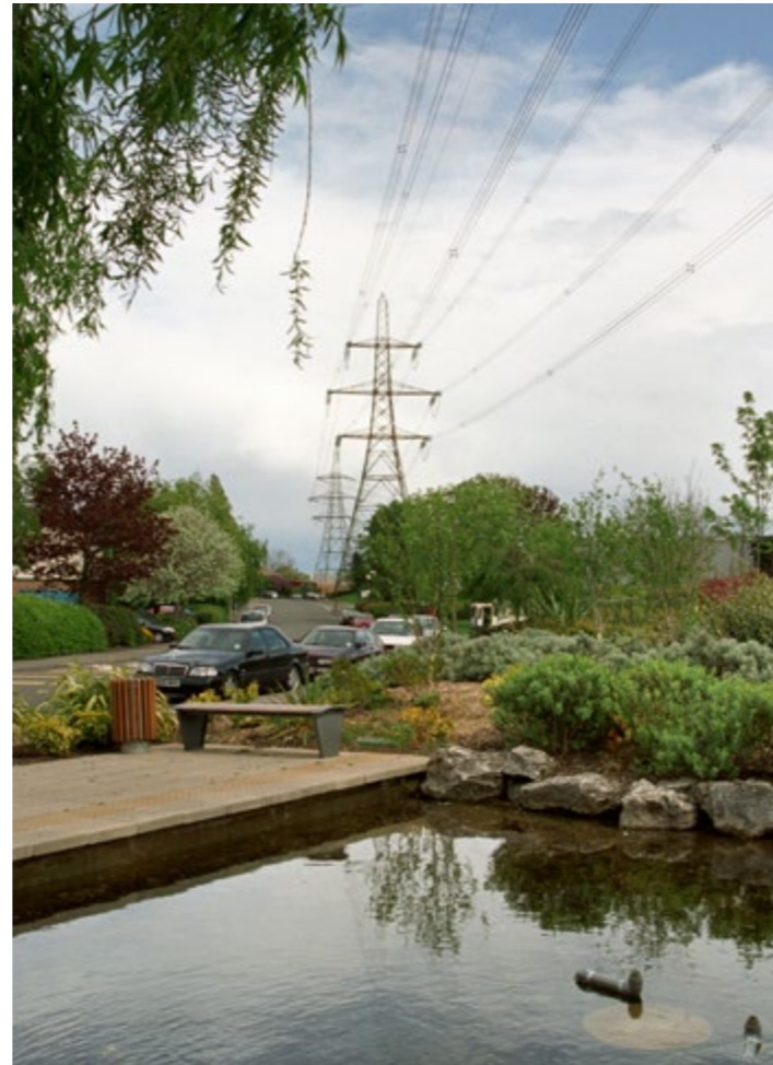
Gravelly Industrial Park, Birmingham—an example of successful commercial development near overhead power lines.
