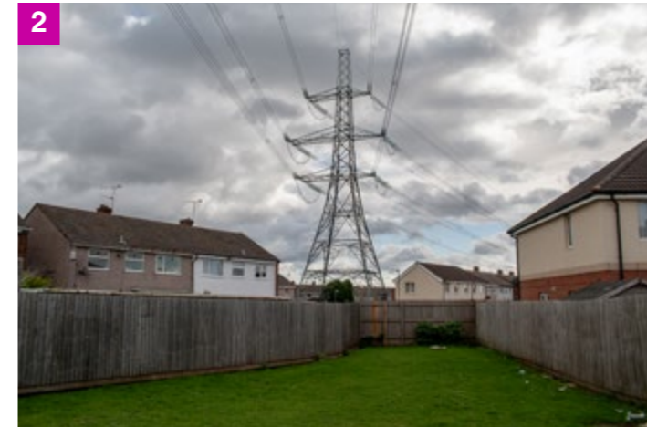
2 The size and shape of the development plot has presented constrained areas of land beneath the overhead lines. While offering little sensory richness, the space does present a degree of opportunity for informal recreational activities.
