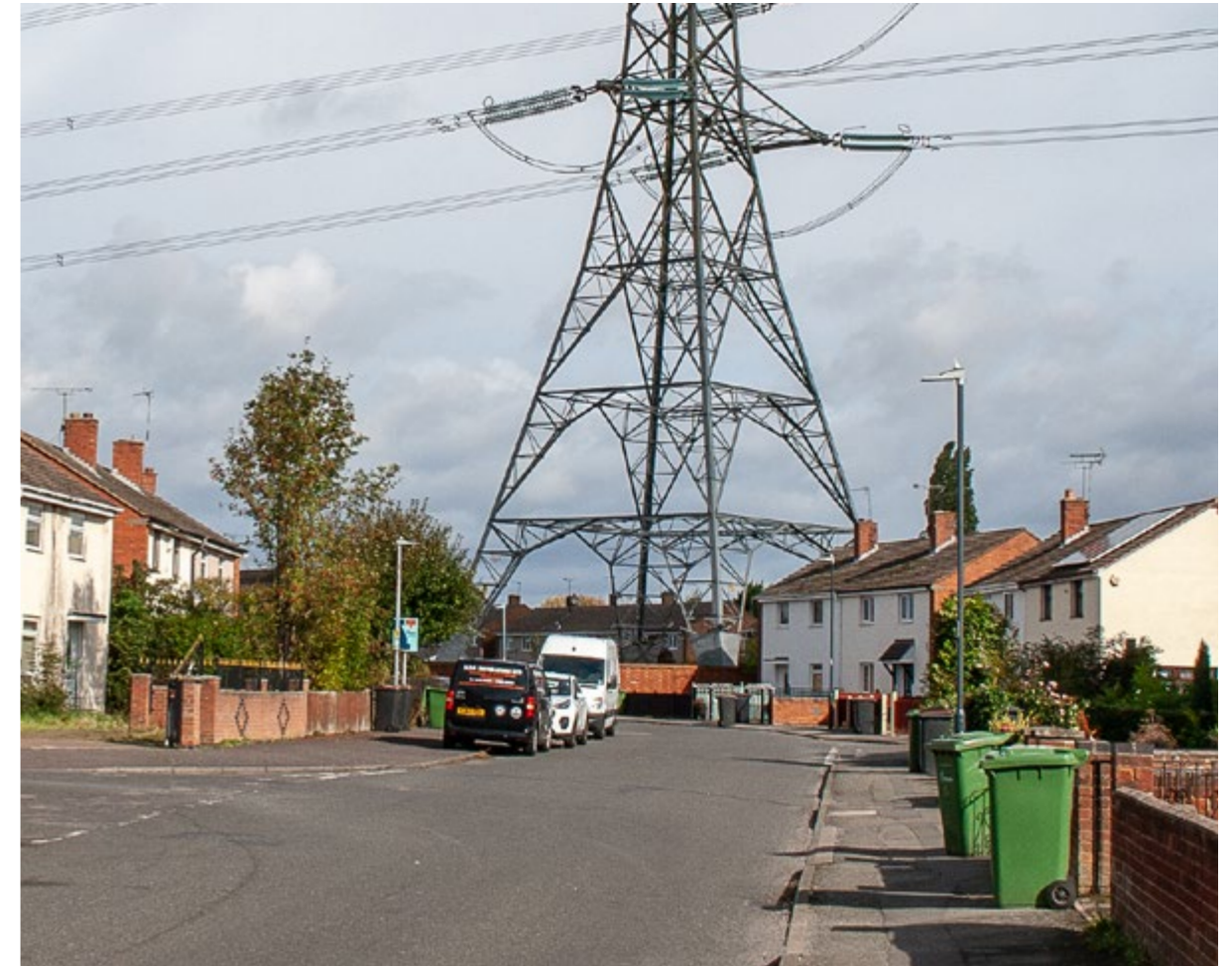
How not to approach the siting of homes near overhead power lines.
