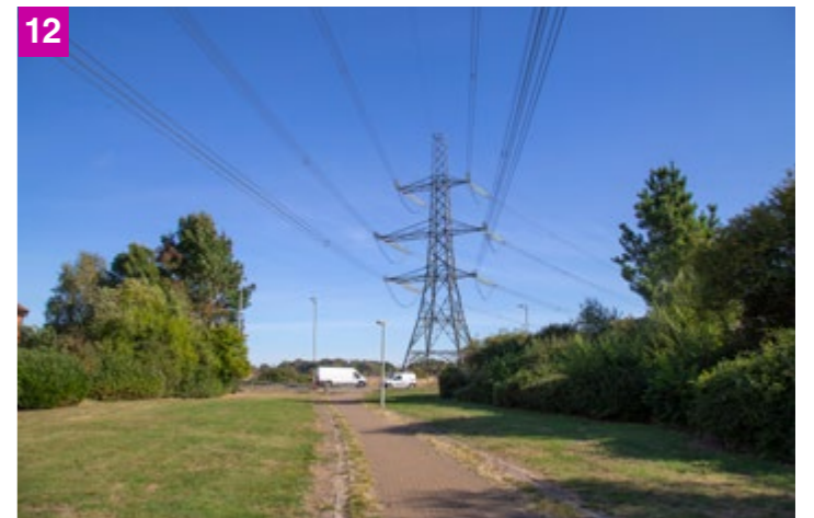
12 The eastern end of the case study ends abruptly. While the linearity of the transmission line is reduced by its change in direction, the lack of planting or public realm treatment leaves a seemingly unfinished end to the open space corridor which is instead defined by the road.
