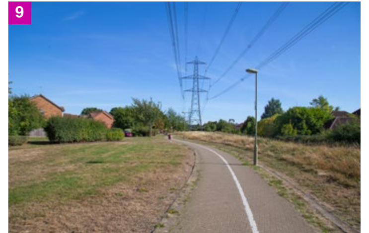
9 The meandering pathway reduces the perceived linearity of the transmission line by changing people's line of sight. The permeable edge allows for visual and physical connectivity to the adjacent housing, thereby offering passive surveillance. The management regime has created formal and informal environments, enhancing sensory richness and the ecological value.
