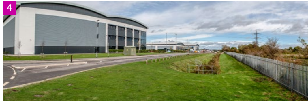
4 A degree of sensory richness is provided by the areas of lawn and tree planting. SUDS are an effective use of the land beneath the transmission line.
