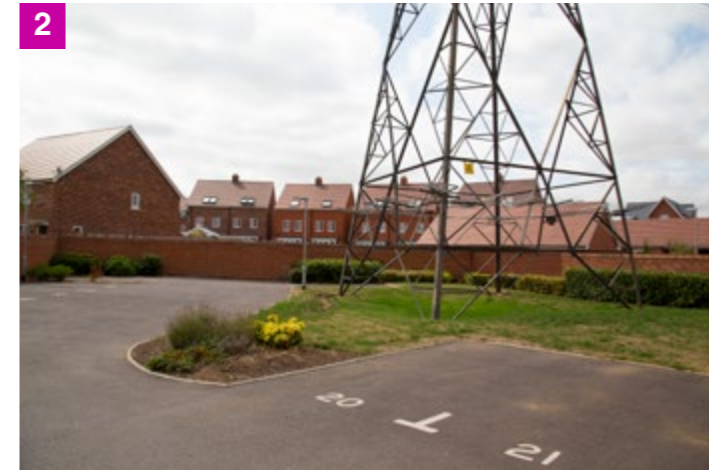
2 Landscaped parking court designed around the base of a pylon, helping to screen views of the structure from surrounding streets and open space.
