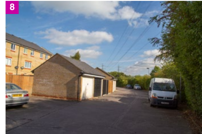
8 The western boundary to the transmission line corridor is defined by a mature tree belt. It provides a degree of effective screening for the adjacent housing however it restricts passive surveillance into the open space and parking areas, presenting a potential security issue. Additionally, the housing backs on to the open space, missing the opportunity to benefit from a park frontage.
