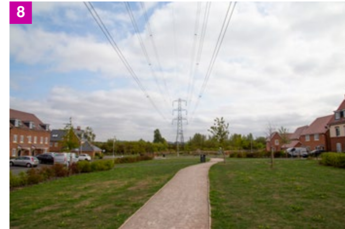
8 The articulated rooflines fronting the space work to reduce the linearity of the transmission line. The mature vegetation in the adjacent Country Park and distant topography work to obscure the base of the pylon, reducing its visual prominence.
