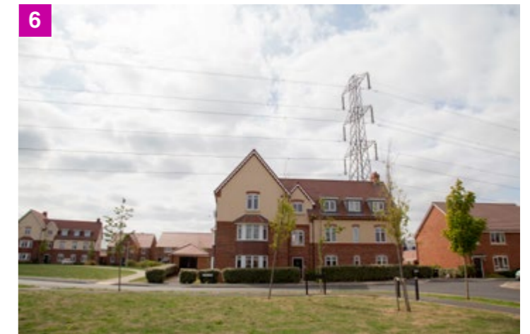
6 Articulation of roofline and building heights provide a focal point for this prominent corner plot and also help to screen views of the pylon base. Once mature, street trees will also contribute to screening while also providing sensory richness.
