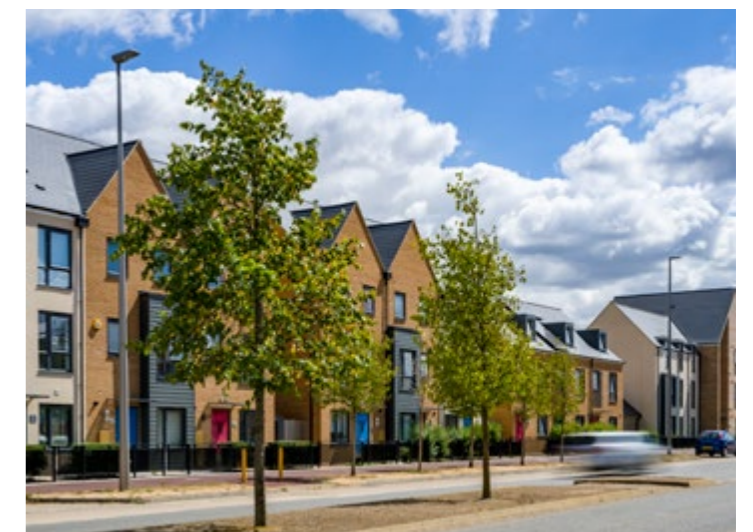
With careful design, a high-quality environment is possible near high voltage overhead lines.
