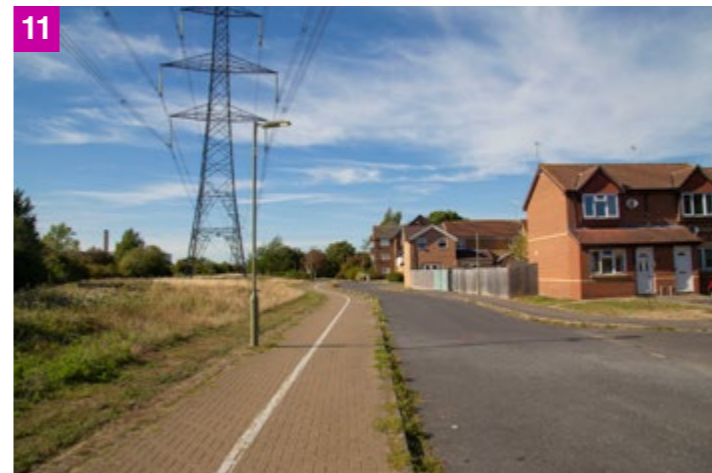
11 The relationship between the adjacent housing and street with the transmission line corridor suffers from a lack of visual and physical connectivity. Road alignment and building orientation run parallel to the overhead lines with fencing and blank facades providing a featureless edge, offering little passive surveillance.
