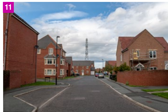
The alignment of the road coincides with the narrowest side profile of the pylon which helps to reduce its visual prominence. The varied roofline helps to reduce the visual prominence of the pylon further by providing a degree of visual distraction.
