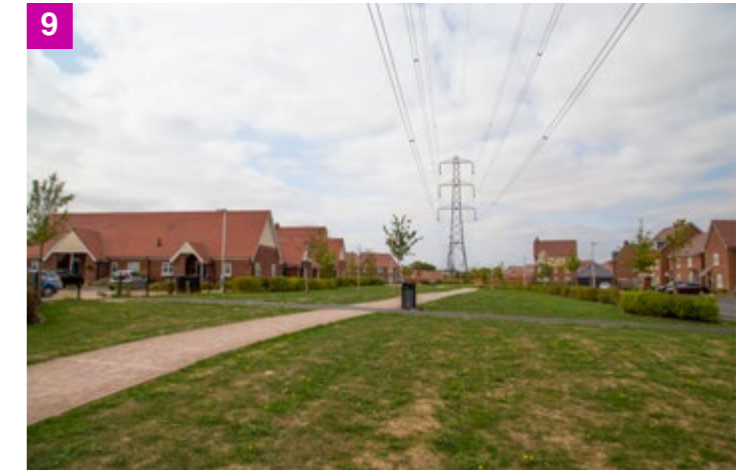
9 The open space is an effective use of land beneath the overhead lines and articulated rooflines and tree planting work to reduce the linearity of the transmission line. However, the raised profile of the open space works to increase visual prominence of the overhead lines as the line of sight is directed upwards as people move through the space.
