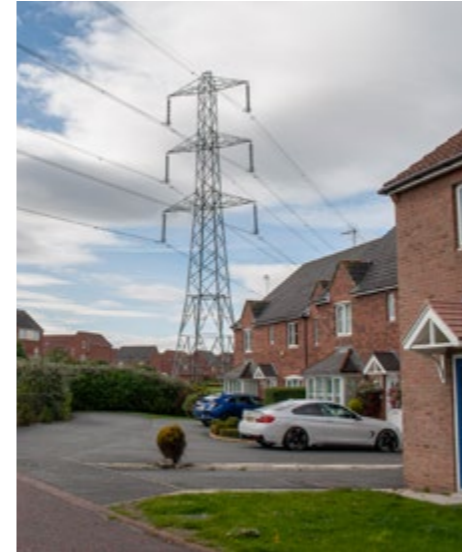
Pylons and lines.
