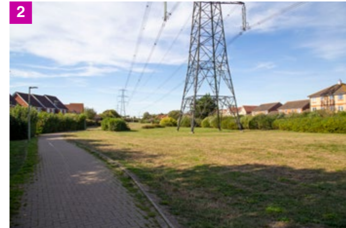
In some locations there is no attempt to provide screening to the pylon structures, as captured in this scenario. The pathway has been designed so as to meander away from the structure, moving people's line of view away and reducing the perceived linearity and prominence of the transmission line.
