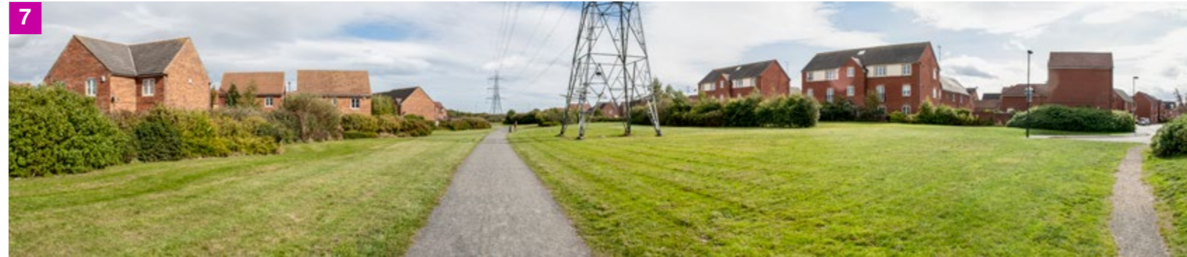
Path connections from the transmission line corridor are limited in places with mature shrub beds creating impermeable edges in places. Desire lines have developed over time as people have established usage patterns. Screening to the pylon structure is limited close to its base, with planting located to the edges instead.
