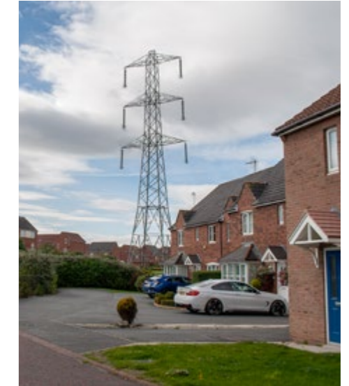
Pylon with lines removed.
