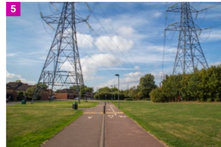
5 Established tree and shrub planting provide a good degree of screening to the base of the pylon to the right, however the lack of planting to the left leaves the structure fully exposed.
