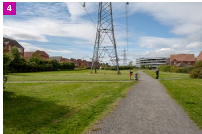
4 Screen planting sits to the edges of the transmission line corridor reducing views of adjacent properties to the pylon structure. Visual prominence of the structure within the open space is strong. The relatively straight path alignment works to emphasise the linearity of the overhead lines.
