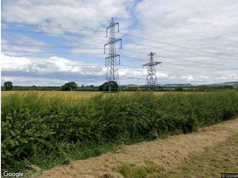
Illustrative wireline image of an overhead line constructed using 'low height' lattice pylons
