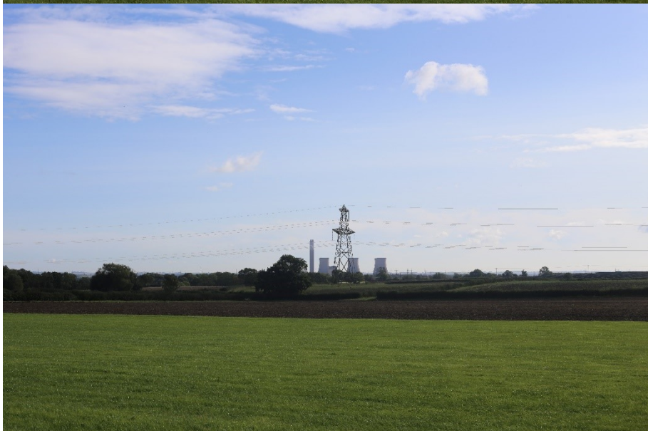
Illustrative wireline image of an overhead line constructed using 'low height' lattice pylons
