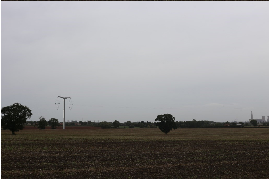
Illustrative wireline image of an overhead line constructed using T-pylon style pylons
