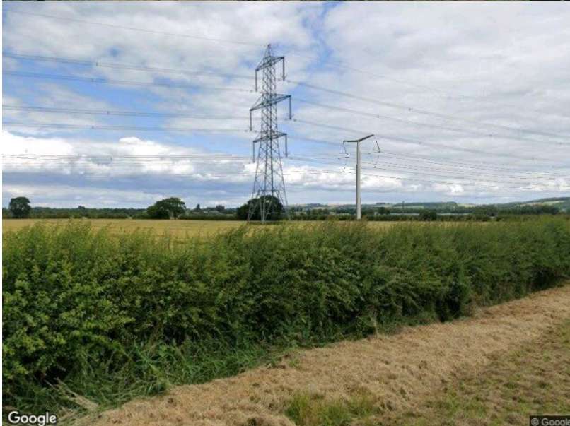
Illustrative wireline image of an overhead line constructed using T-pylon style pylons
