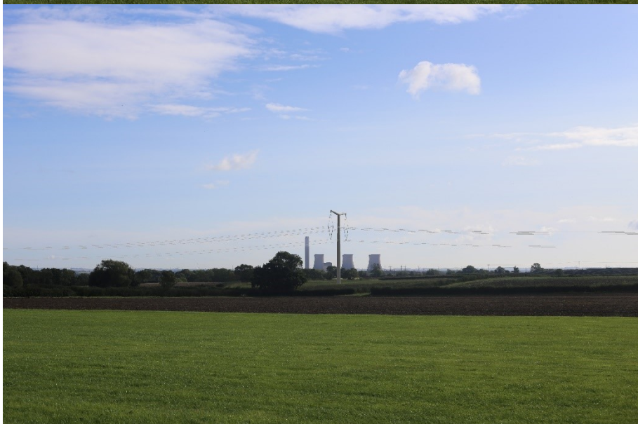
Illustrative wireline image of an overhead line constructed using T-pylon style pylons
