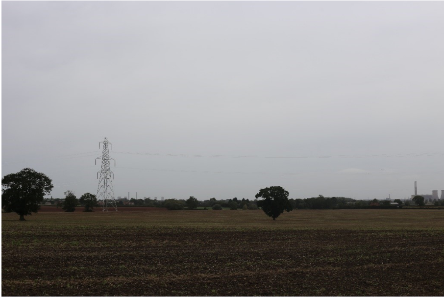
Illustrative wireline image of an overhead line constructed using the standard lattice pylon
