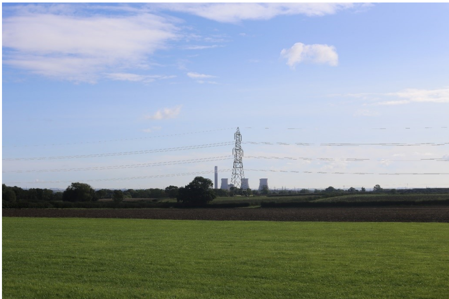
Illustrative wireline image of an overhead line constructed using the standard lattice pylon
