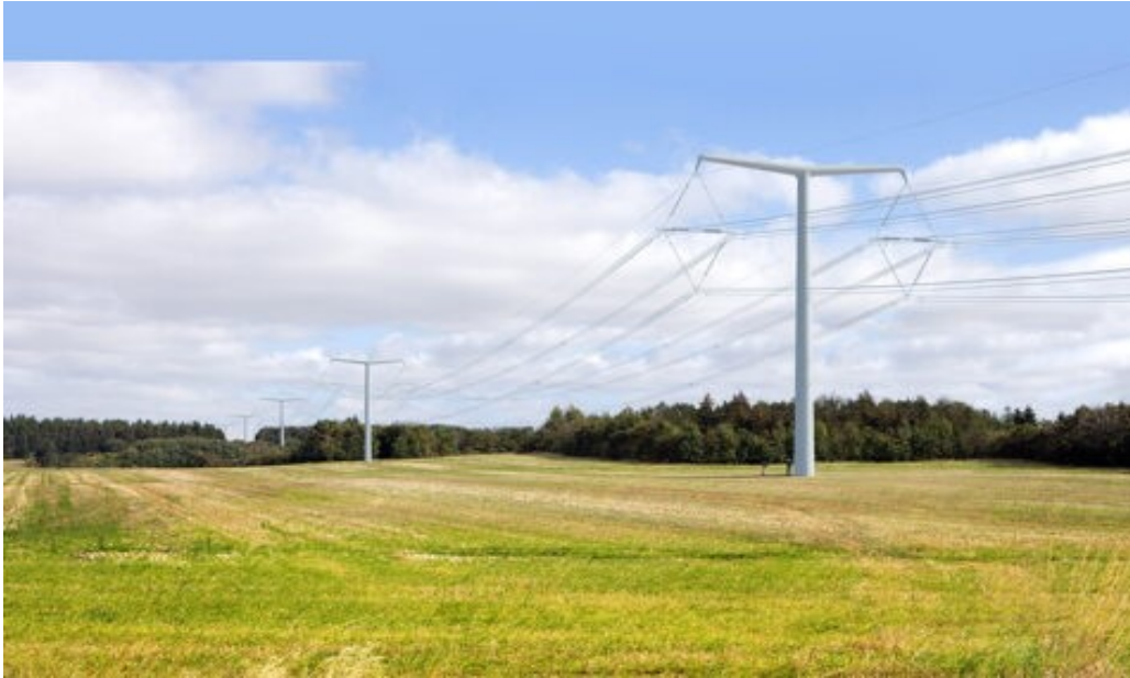
Figure C.2 – The T-pylon
