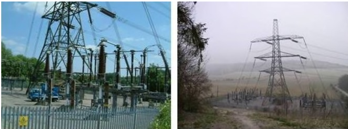
Figure C.5 – Cable Sealing End Compounds
