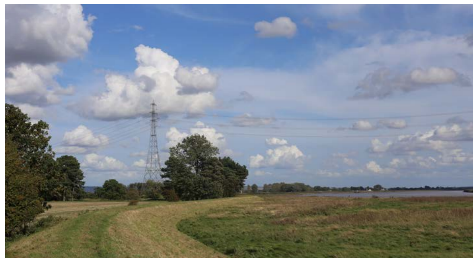
The existing 400 kV overhead line crossing the River Ouse from the Trans Pennine Trail
