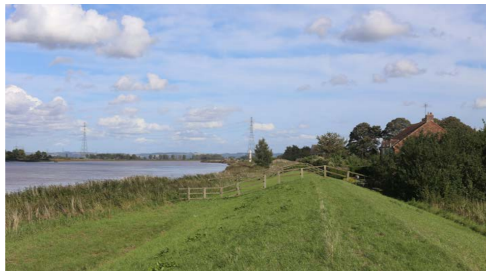
Extensive views from the embankments along the River Ouse, the existing 400 kV overhead line visible to the east
