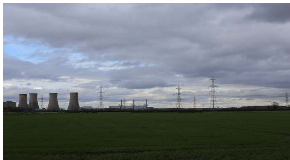
Former power stations and overhead lines are defining features of this RLCT
