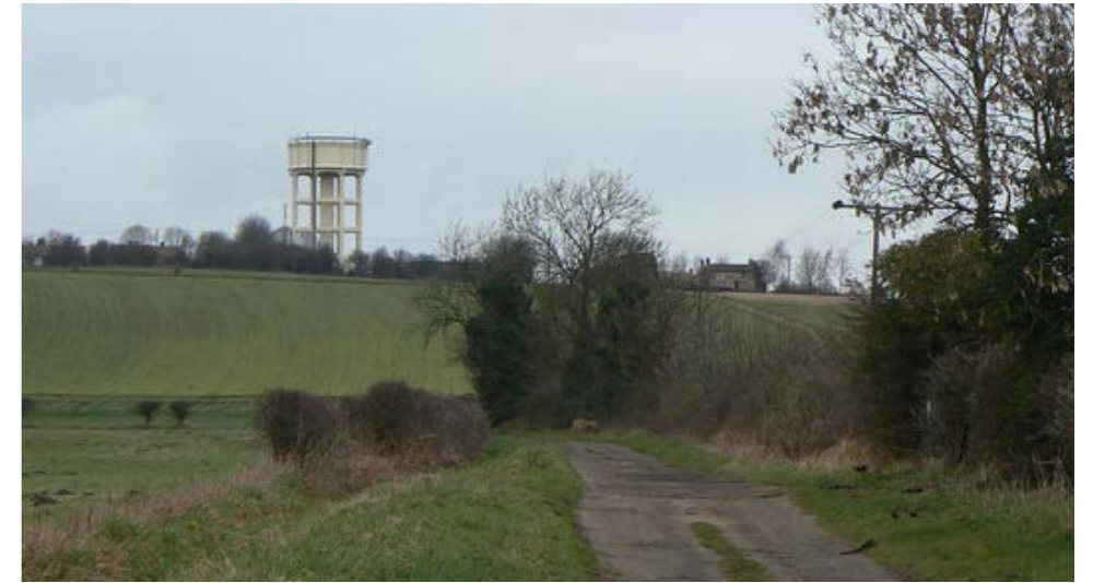
The water tower at Haxey is a prominent feature on elevated landform Photo © Alan Murray-Rust (cc-by-sa/2.0)
