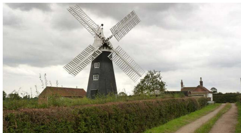
North Leverton Windmill remains a working mill with small museum located to the west of North Leverton with Hablesthorpe
