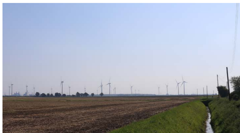
Keadby Windfarm with Keadby Substation on the skyline
