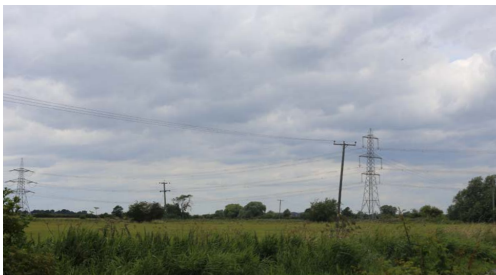
This existing 400 kV overhead line is a feature to the east of the LCT
